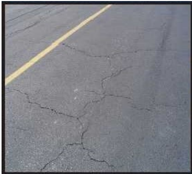
Figure A-10 Medium-Severity Block Cracking
