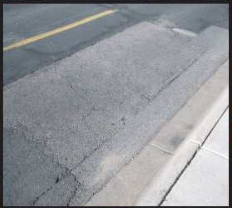
Figure A-43 Medium-Severity Patch and Utility Cut Patching
