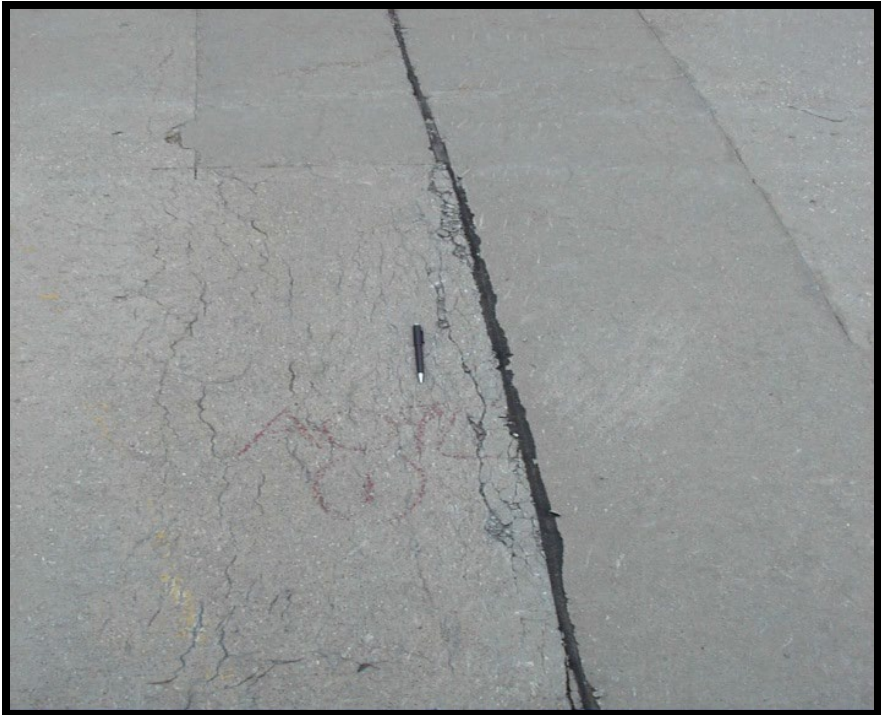
Figure A-240 High-Severity "D" Cracking
