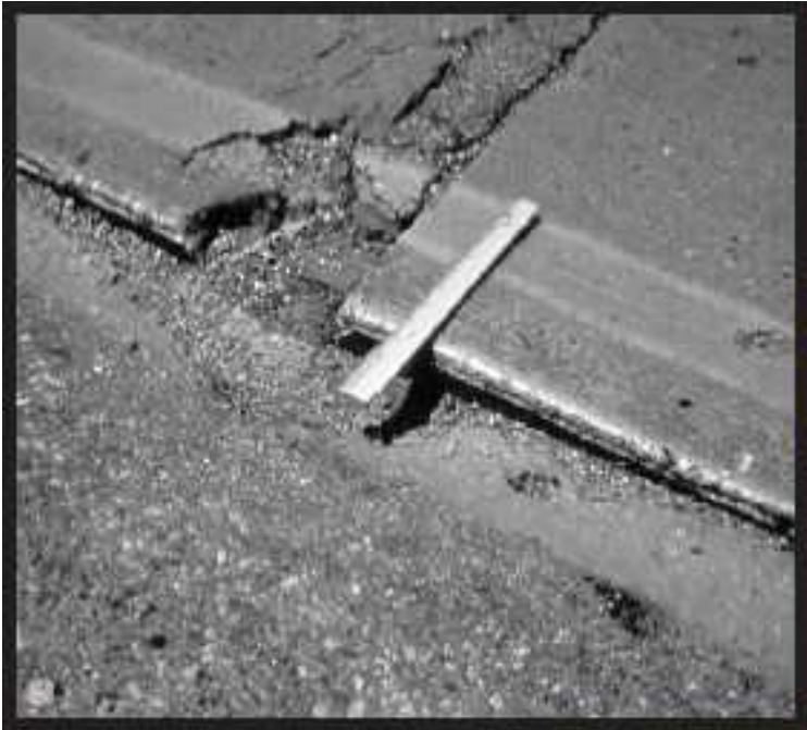
Figure A-103 Medium-Severity Lane/Shoulder Drop-off
