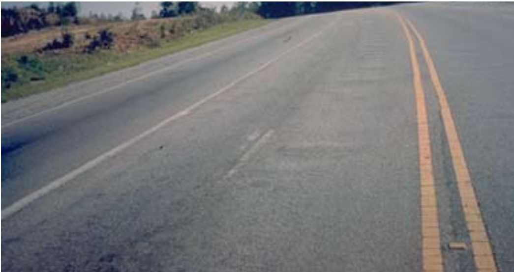
Figure A-164 Medium-Severity Corrugation
