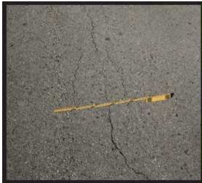
Figure A-2 Medium-Severity Alligator Cracking
