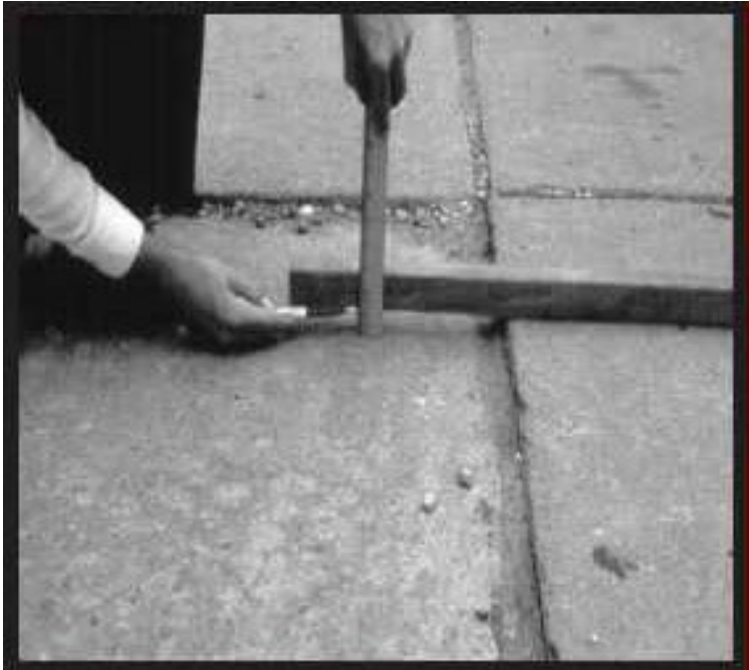
Figure A-96 High-Severity Faulting
