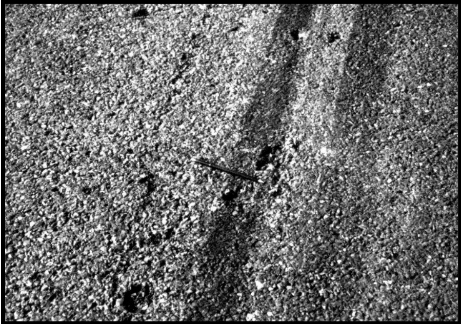
Figure A-203 High-Severity Raveling (PFC)
