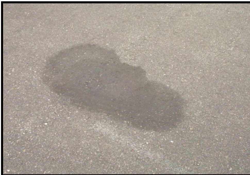
Figure A-186 Oil Spillage
