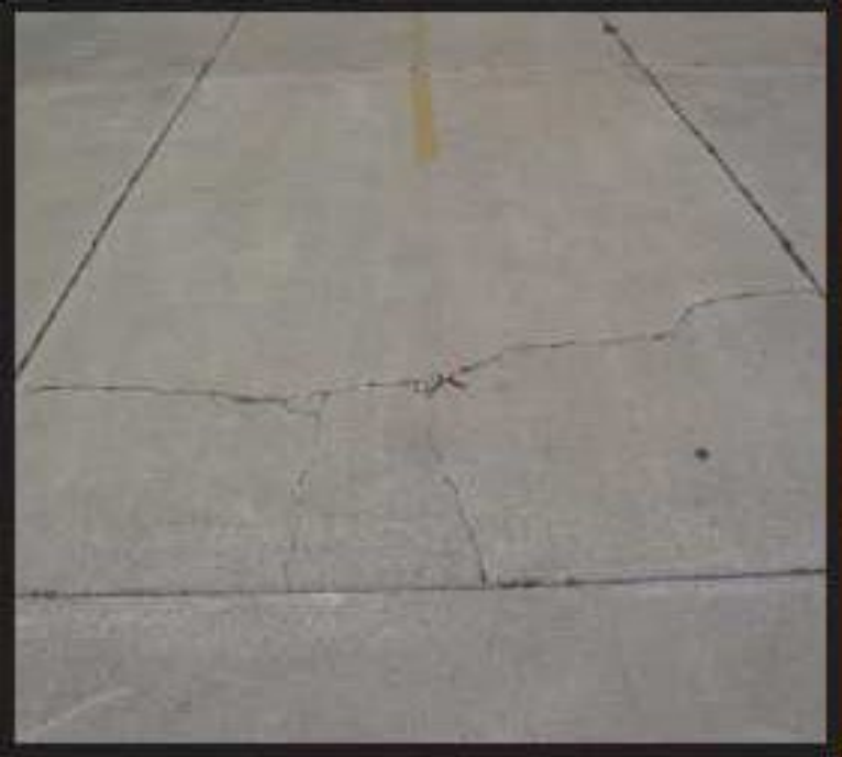
Figure A-126 Medium-Severity Punchout
