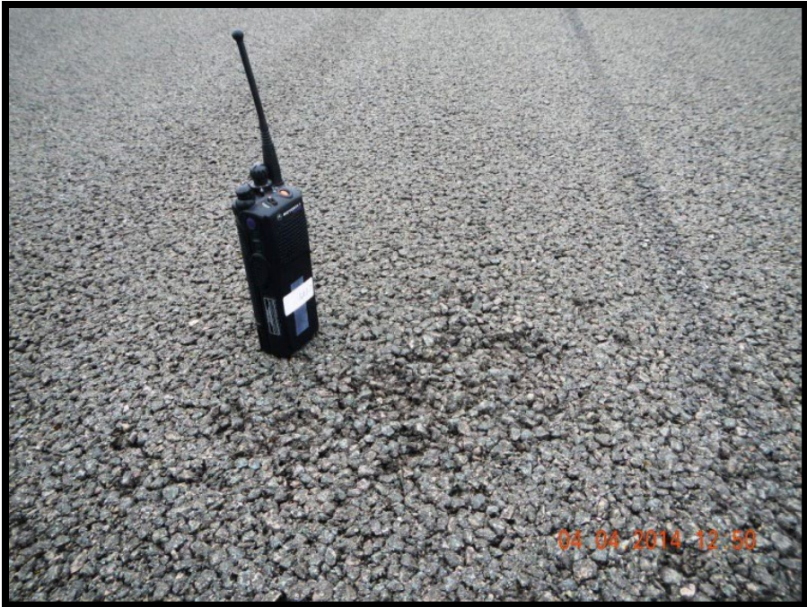
Figure A-203 High-Severity Raveling (PFC)
