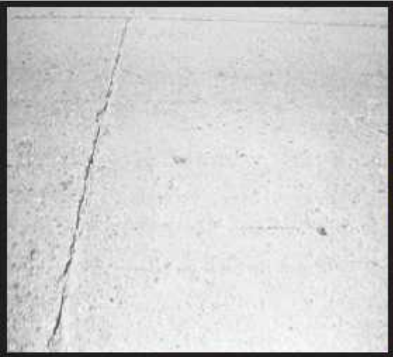
Figure A-144 Medium-Severity Joint Spall
