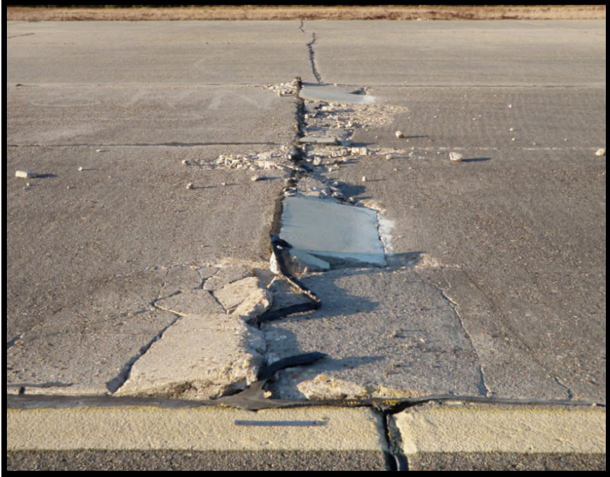
Figure A-227 High-Severity Blowup
