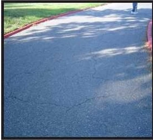
Figure A-10 Medium-Severity Block Cracking
