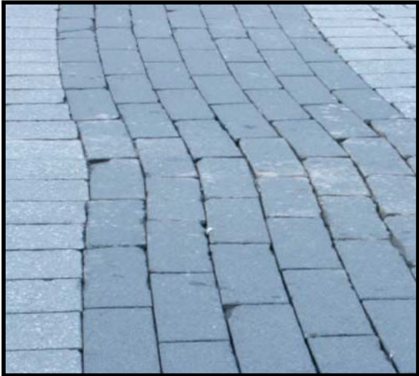
Figure A-326 High Severity Horizontal Creep
