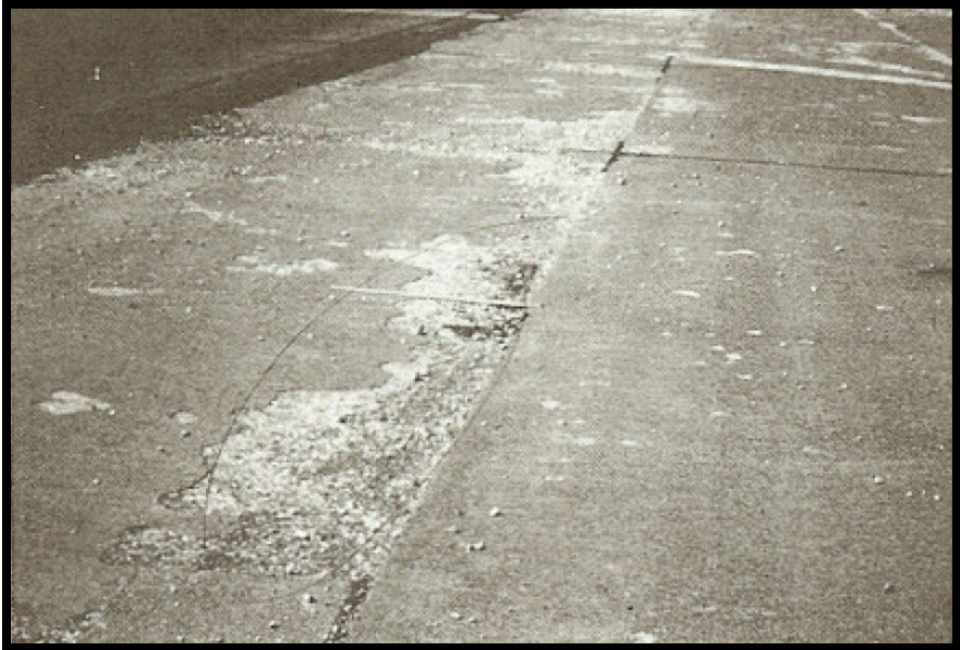
Figure A-261 High-Severity Scaling
