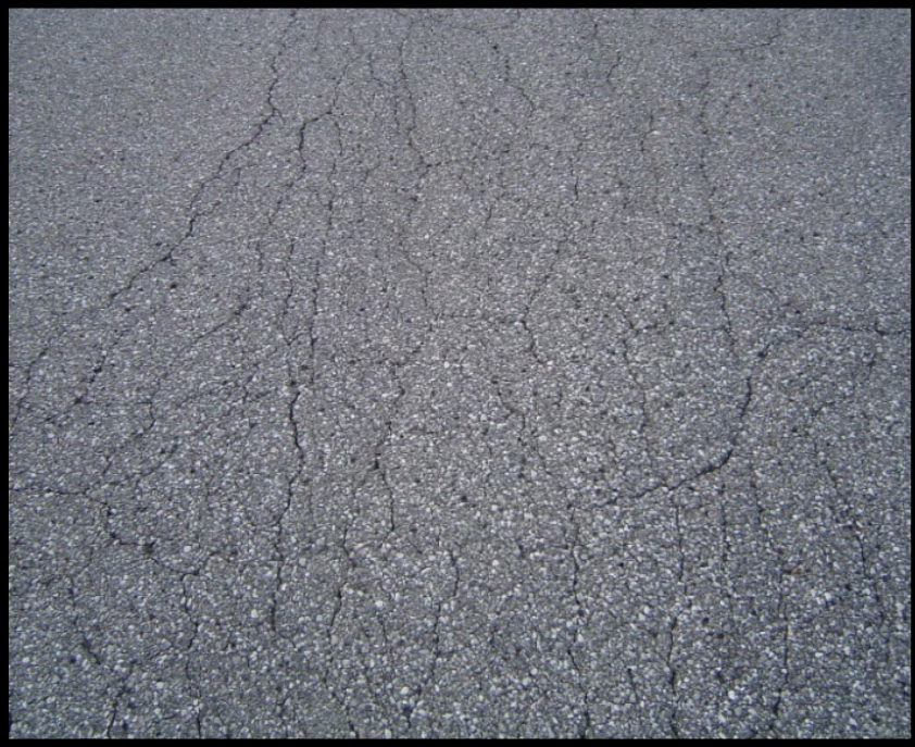
Figure A-149 Medium-Severity Alligator Cracking
