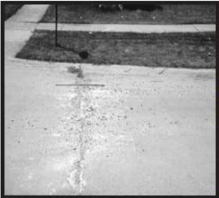
Figure A-79 Medium-Severity Blowup/Buckling
