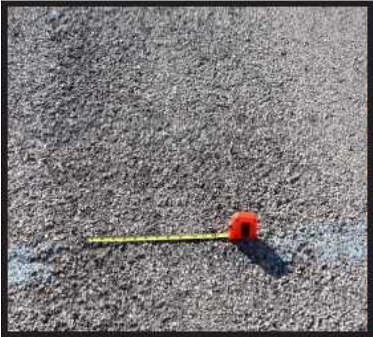
Figure A-71 High-Severity Raveling
