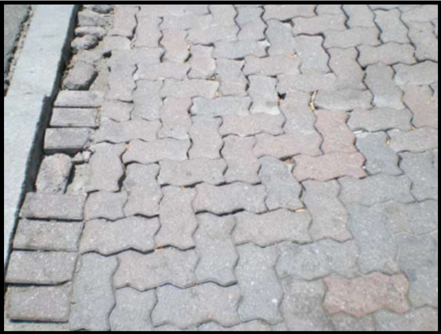
Figure A-310 High-Severity Edge Restraint Damage
