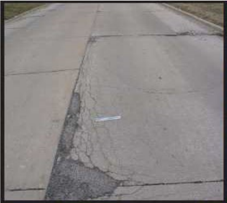
Figure A-91 Medium-Severity Durability Cracking
