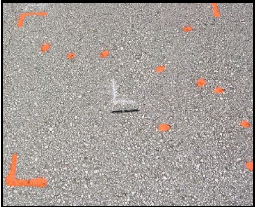
Figure A-195 Medium-Severity Raveling (Dense Mix)
