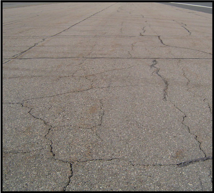
Figure A-158 Medium-Severity Block Cracking
