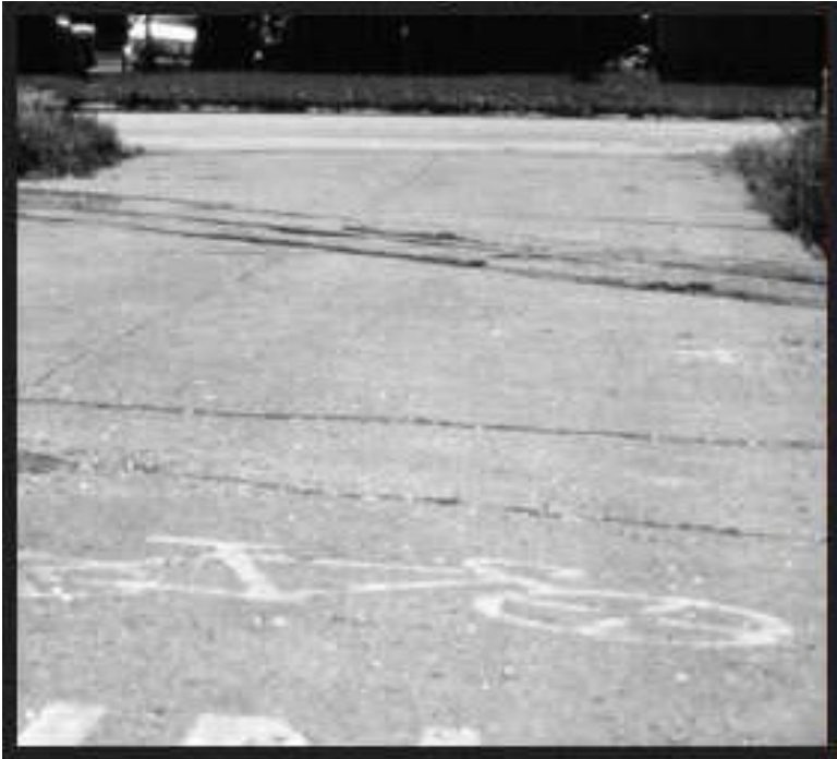
Figure A-131 High-Severity Railroad Crossing
