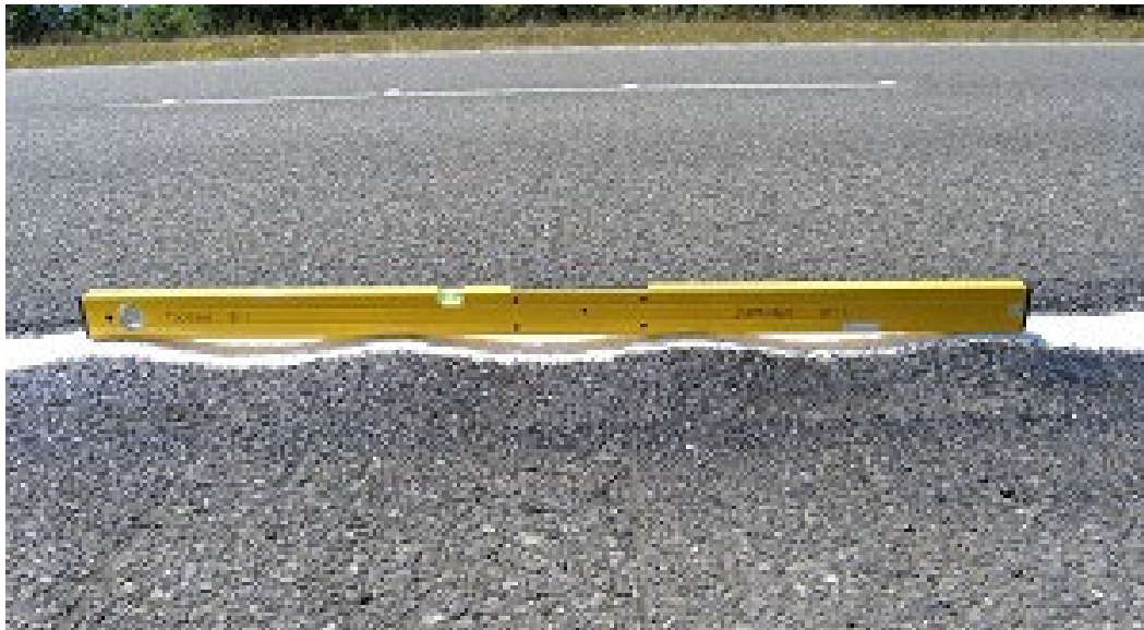
Figure A-164 Medium-Severity Corrugation
