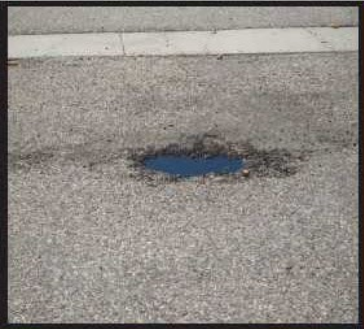
Figure A-50 High-Severity Pothole
