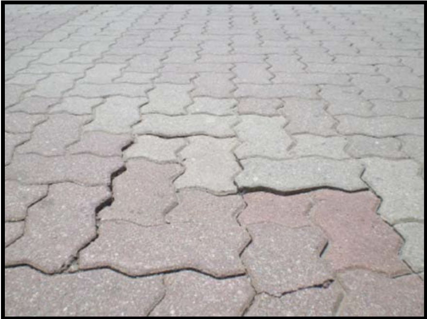
Figure A-318 High-Severity Faulting
