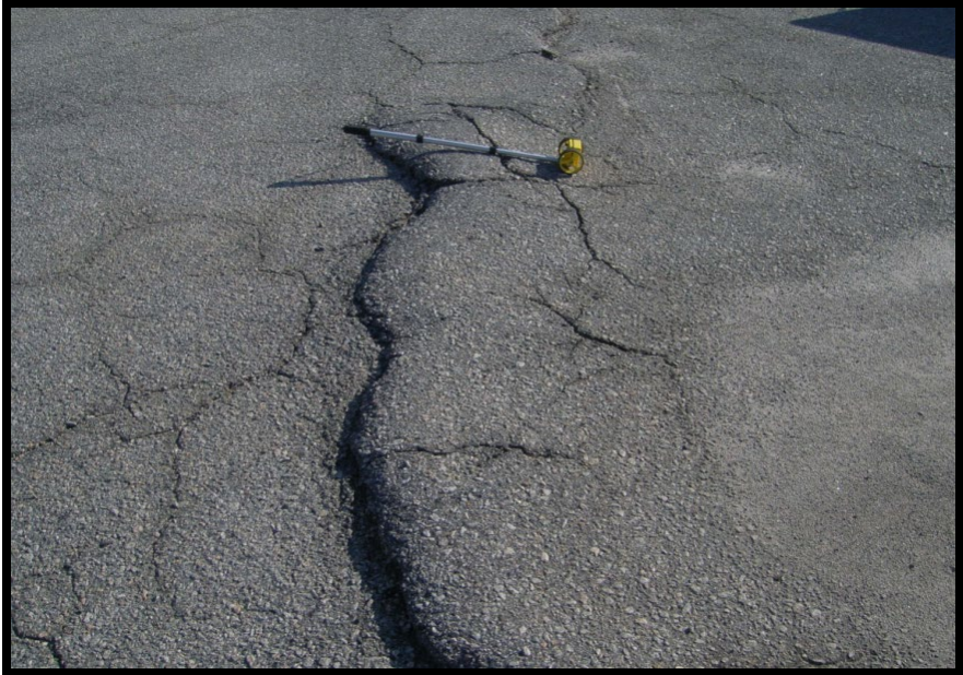
Figure A-217 High-Severity Swell
