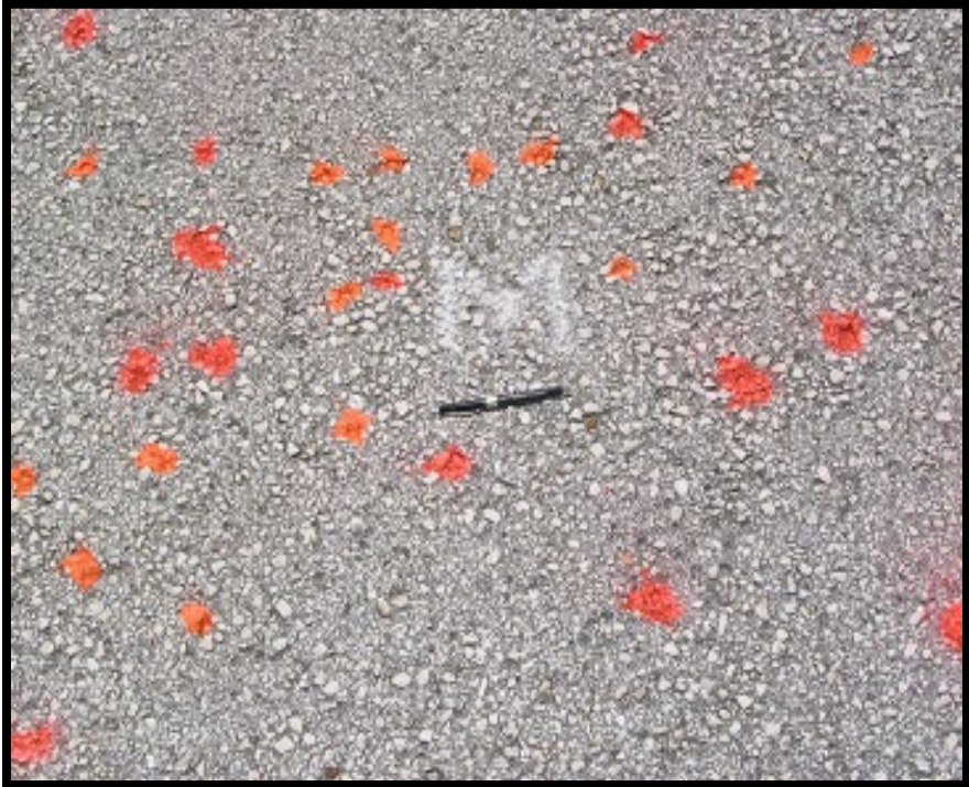
Figure A-195 Medium-Severity Raveling (Dense Mix)
