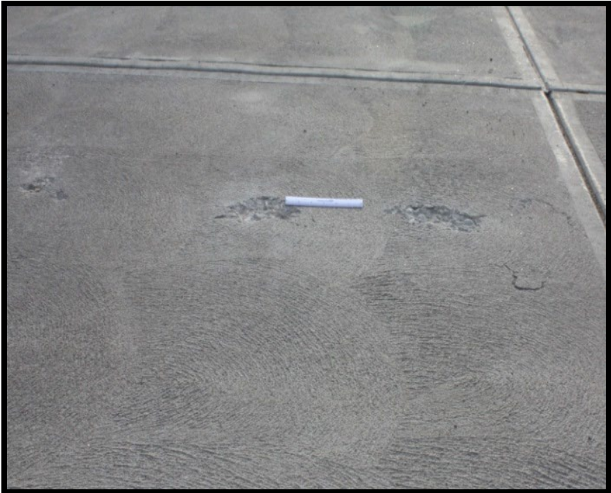
Figure A-261 High-Severity Scaling
