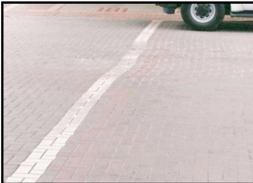
Figure A-305 Medium-Severity Depression
