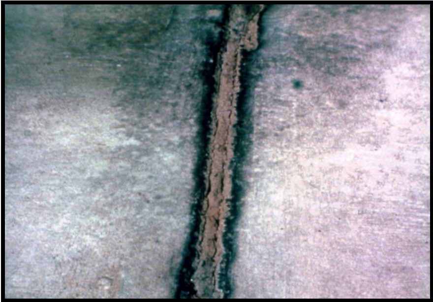
Figure A-257 Pumping Stains
