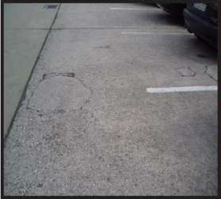
Figure A-115 Medium-Severity Small Patch
