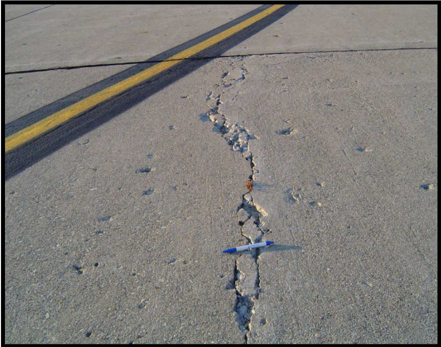
Figure A-235 High-Severity Linear Cracking
