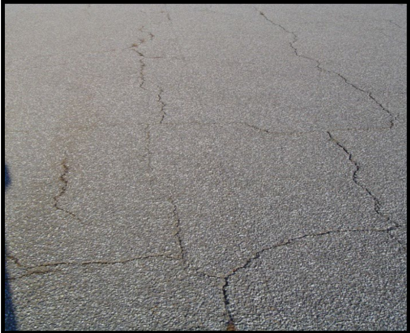
Figure A-158 Medium-Severity Block Cracking
