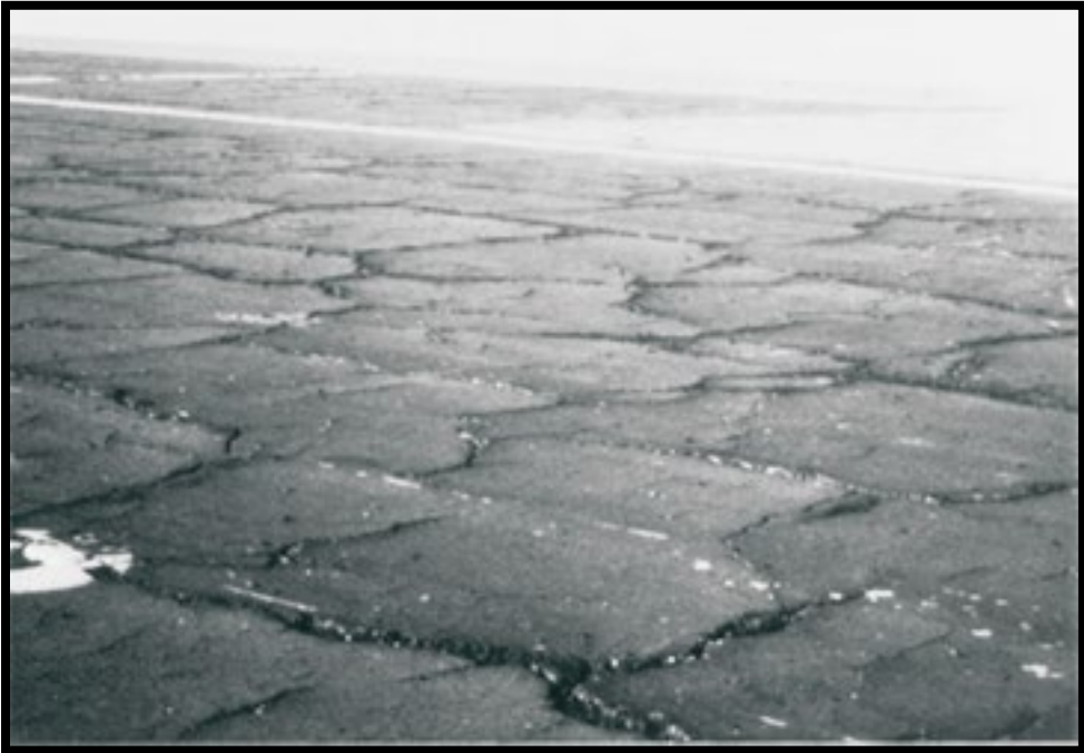
Figure A-160 High-Severity Block Cracking
