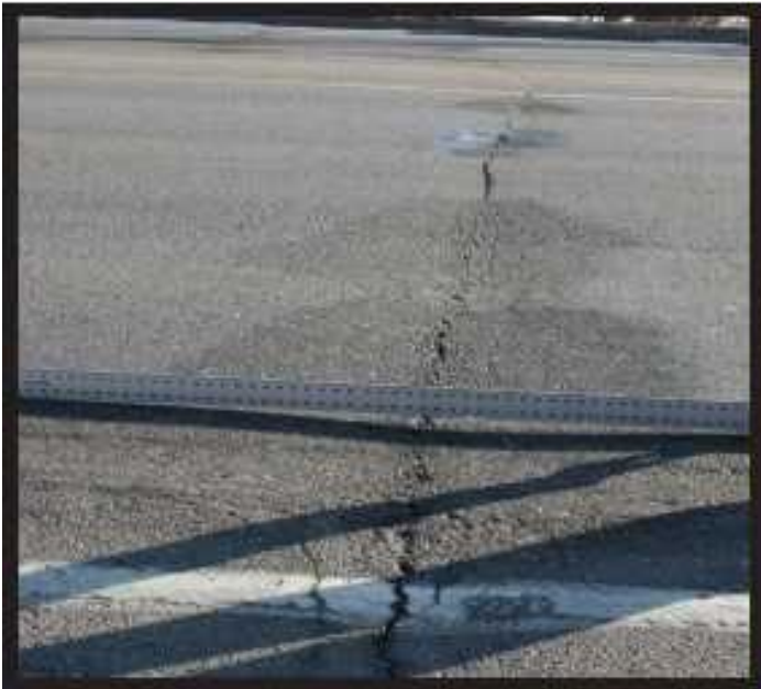
Figure A-14 Medium-Severity Bump or Sag
