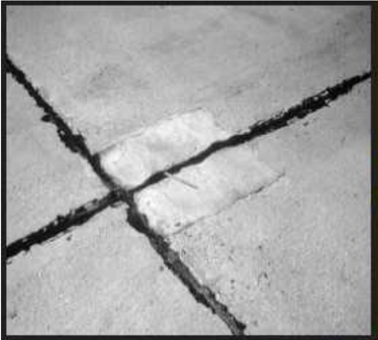
Figure A-115 Medium-Severity Small Patch
