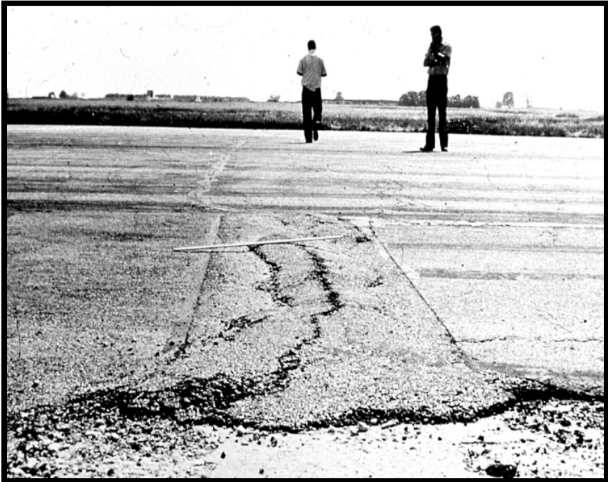
Figure A-190 High-Severity Patching
