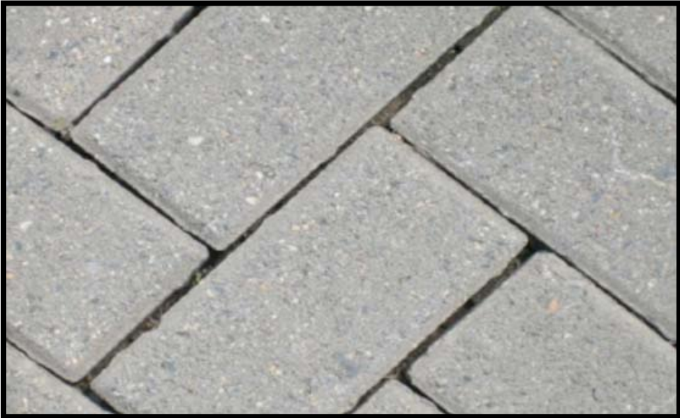
Figure A-329 Medium-Severity Joint Sand Loss
