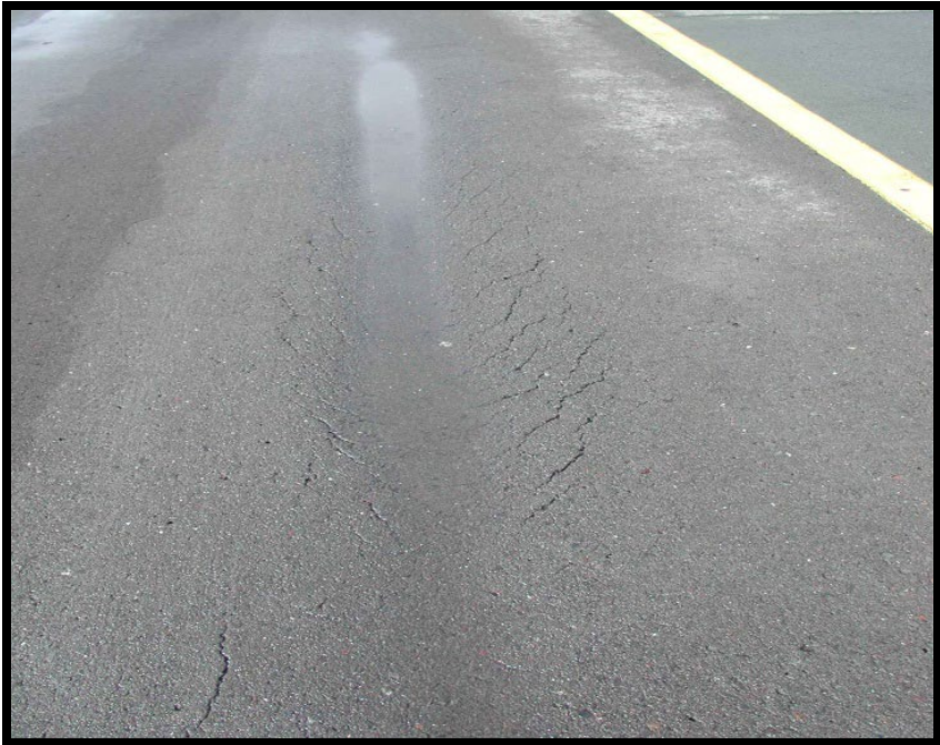
Figure A-207 High-Severity Rutting
