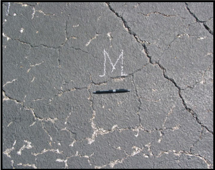
Figure A-198 Medium-Severity Raveling (Slurry Seal/Coal Tar Over Dense Mix)
