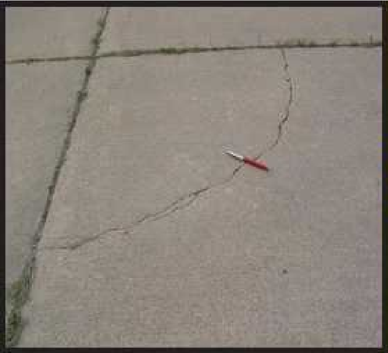
Figure A-83 Medium-Severity Corner Break
