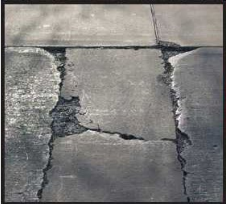
Figure A-112 High-Severity Large Patch and Utility Cut
