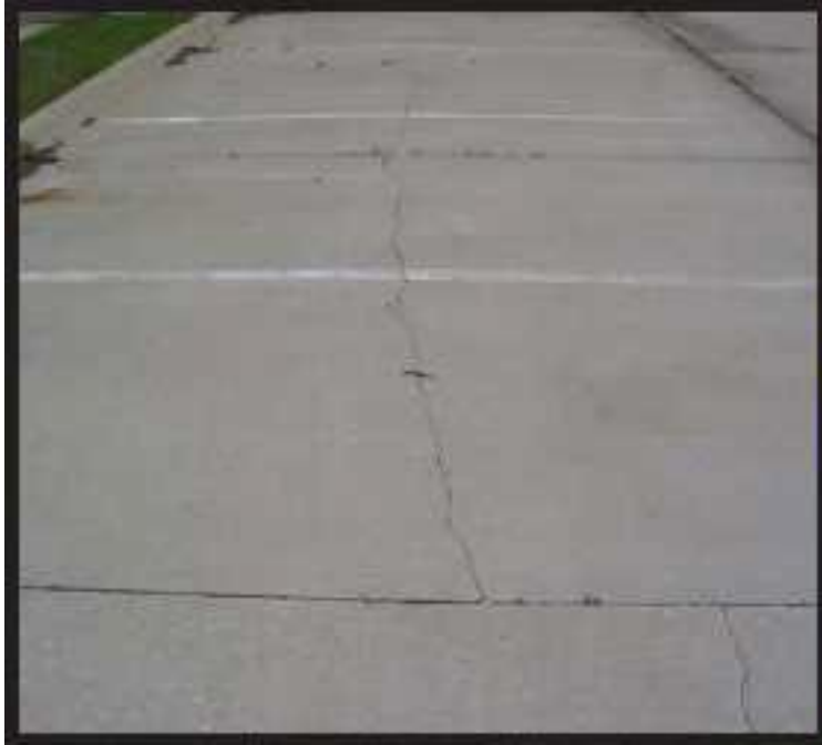
Figure A-107 Medium-Severity Linear Cracking
