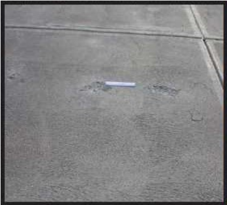
Figure A-134 Medium-Severity Scaling
