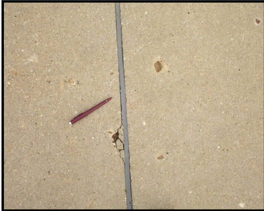
Figure A-274 Medium-Severity Joint Spall
