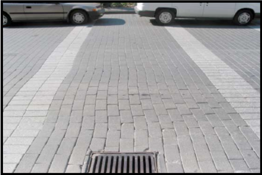
Figure A-326 High Severity Horizontal Creep
