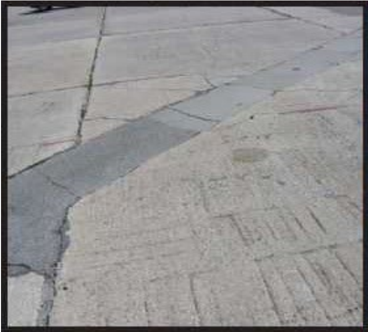
Figure A-112 High-Severity Large Patch and Utility Cut
