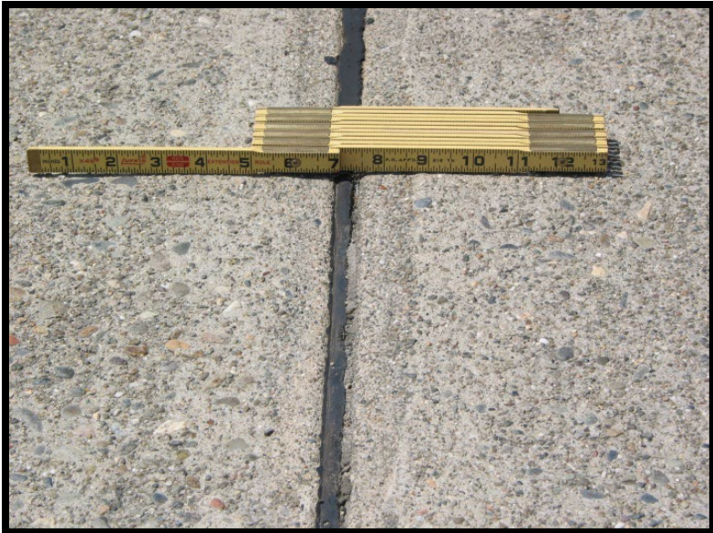
Figure A-243 Medium-Severity Joint Seal Damage
