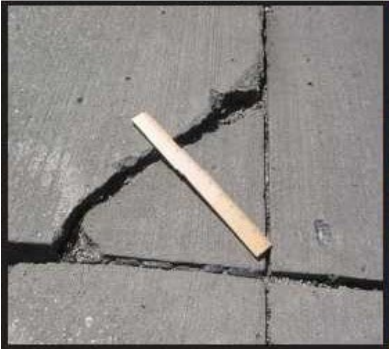
Figure A-141 High-Severity Corner Spall
