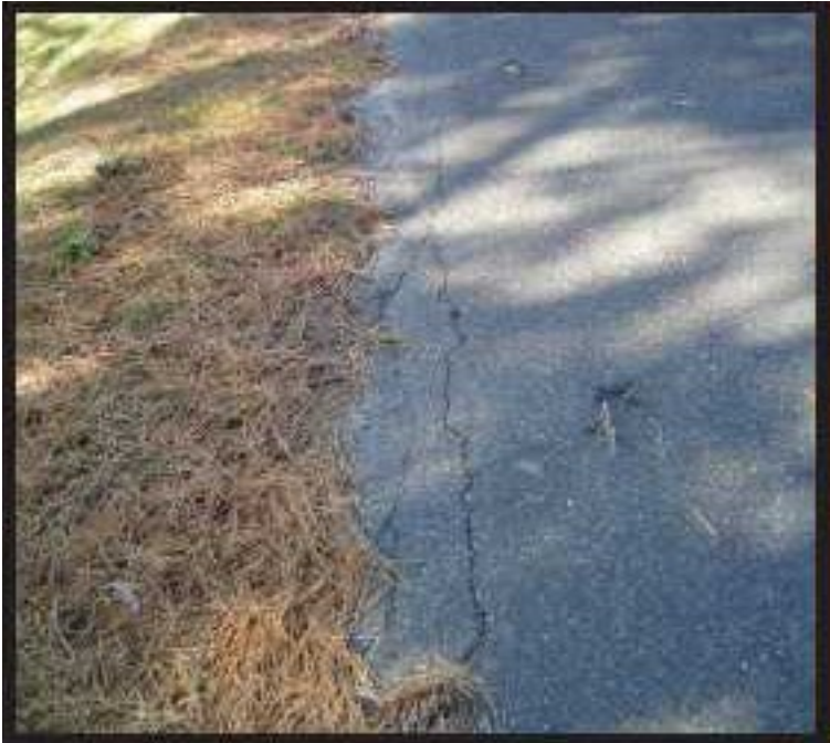
Figure A-27 Medium-Severity Edge Cracking
