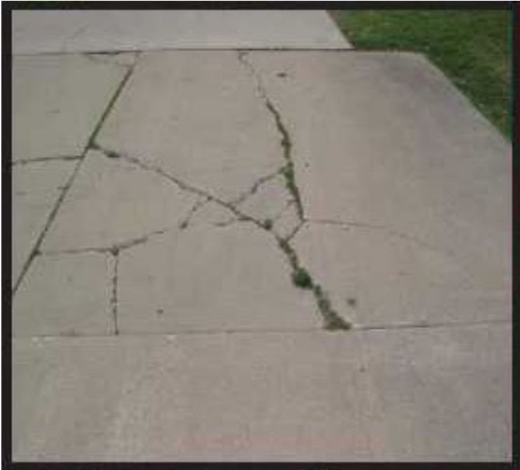
Figure A-88 High-Severity Divided Slab
