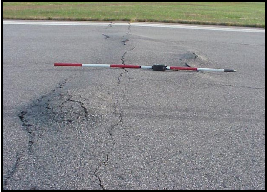
Figure A-217 High-Severity Swell
