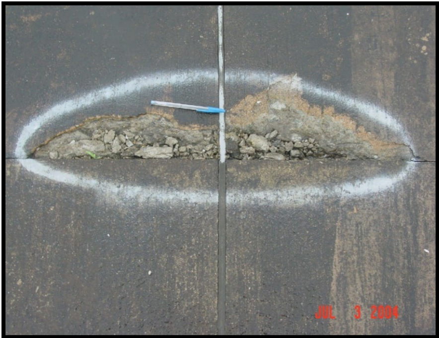
Figure A-276 High-Severity Joint Spall
