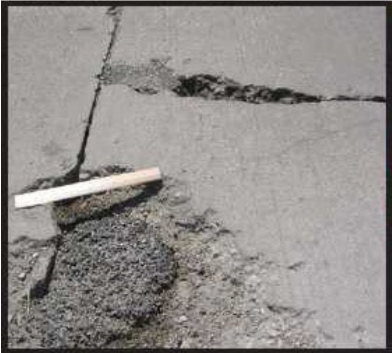
Figure A-141 High-Severity Corner Spall
