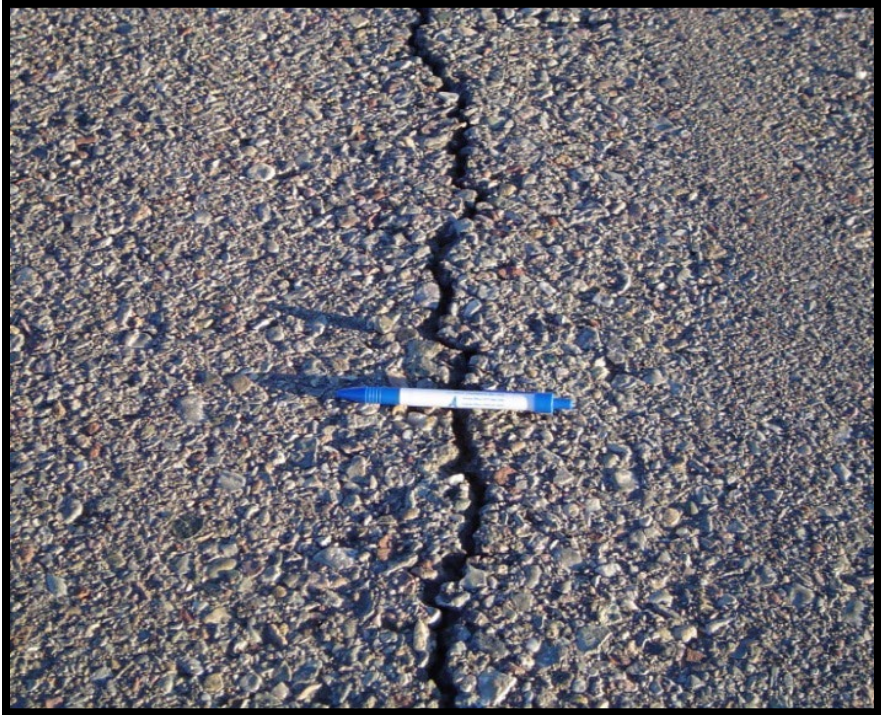
Figure A-179 Medium-Severity L&T Cracking
