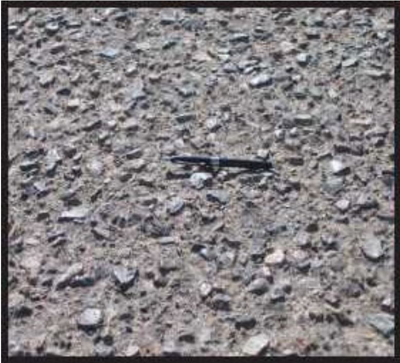
Figure A-75 High-Severity Weathering
