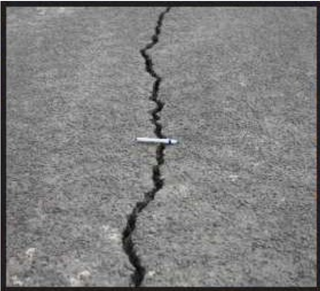
Figure A-39 Medium-Severity Longitudinal and Transverse Cracking
