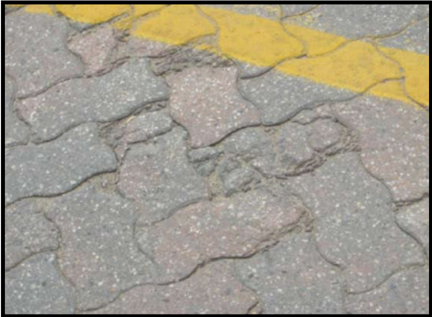
Figure A-302 High-Severity Damaged Pavers
