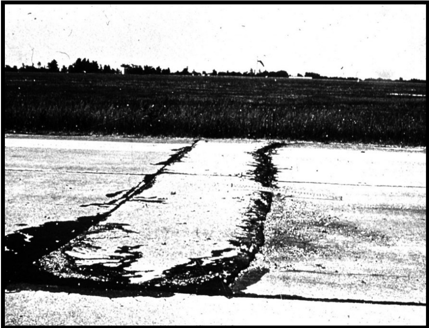
Figure A-227 High-Severity Blowup
