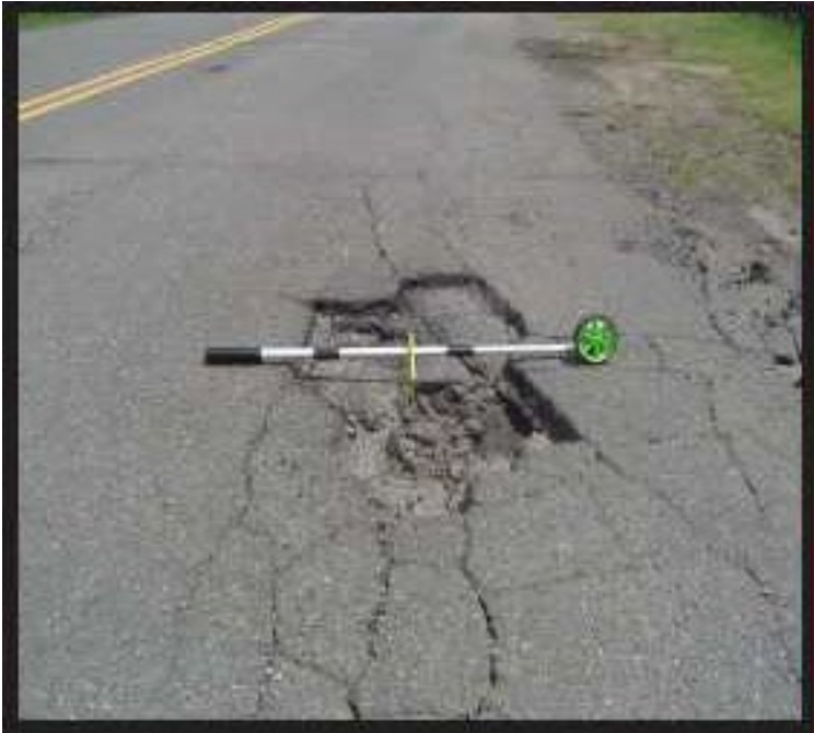
Figure A-50 High-Severity Pothole
