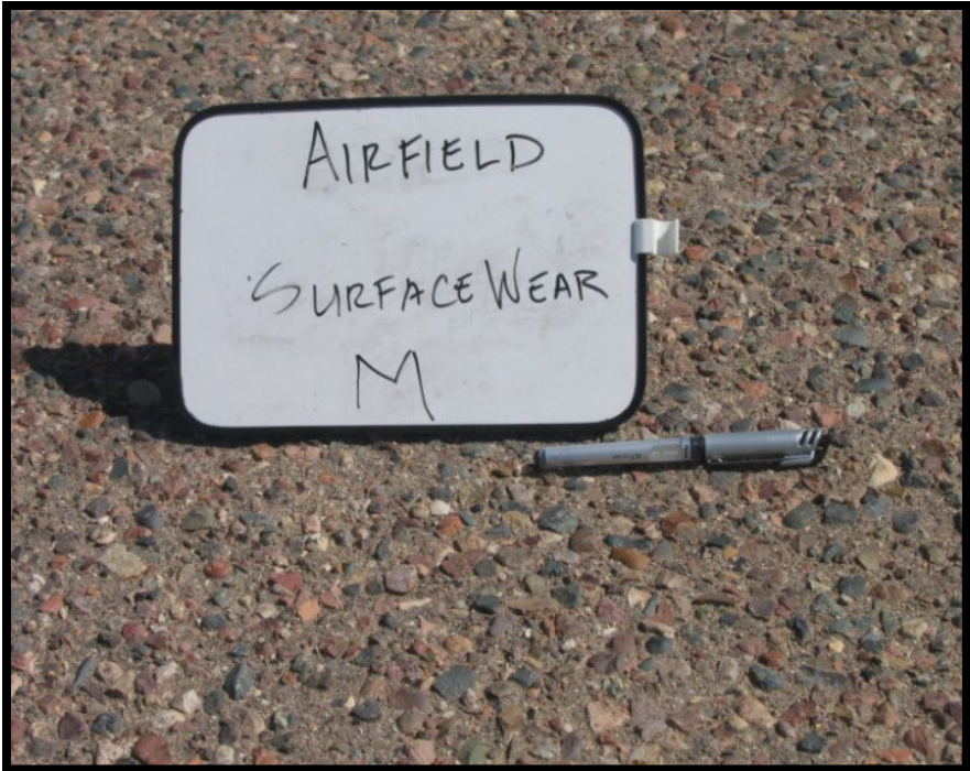
Figure A-221 High-Severity Weathering
