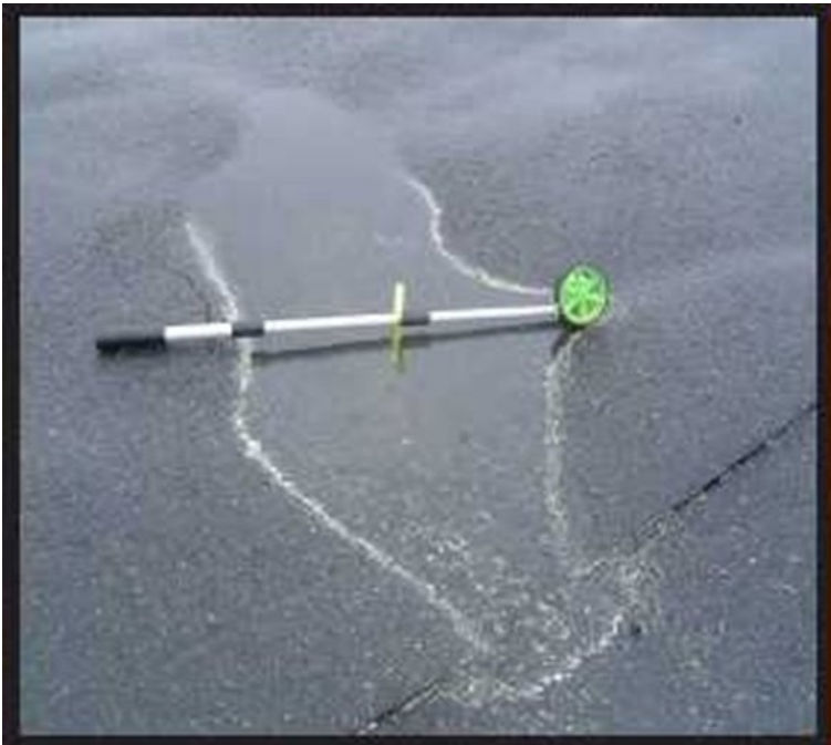
Figure A-24 High-Severity Depression
