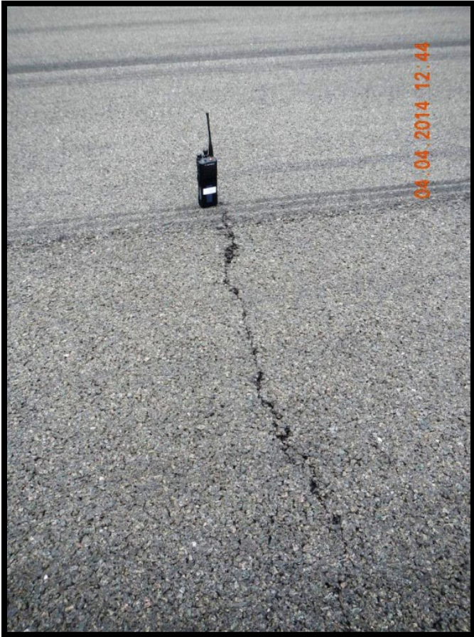
Figure A-183 Medium-Severity PFC L&T Cracking
