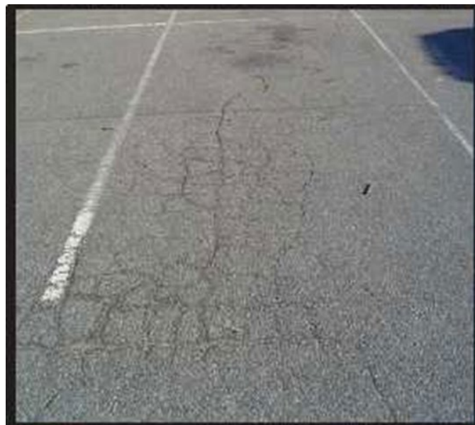
Figure A-2 Medium-Severity Alligator Cracking
