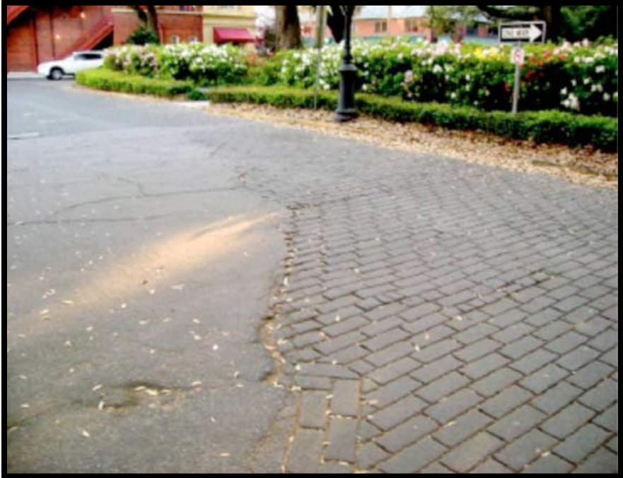
Figure A-337 Medium-Severity Patch
