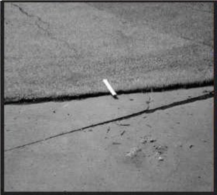
Figure A-62 High-Severity Shoving
