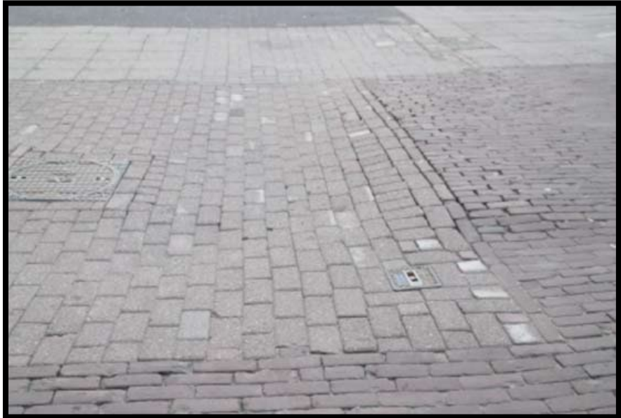
Figure A-321 Medium-Severity Heave
