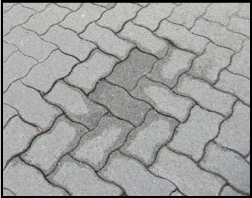
Figure A-313 Medium-Severity Excessive Joint Width
