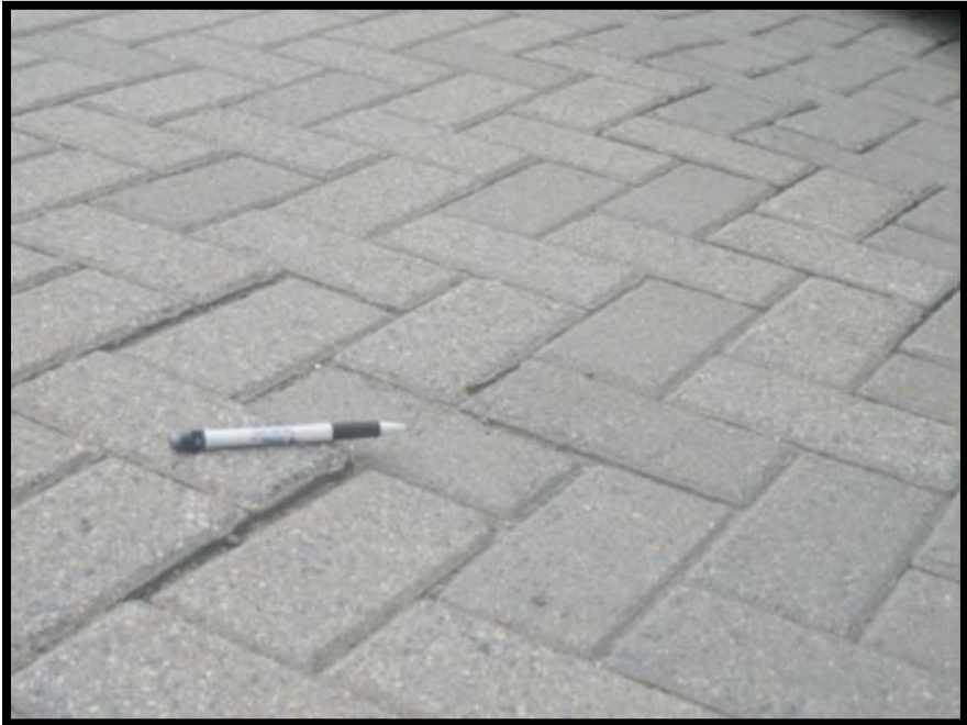
Figure A-318 High-Severity Faulting
