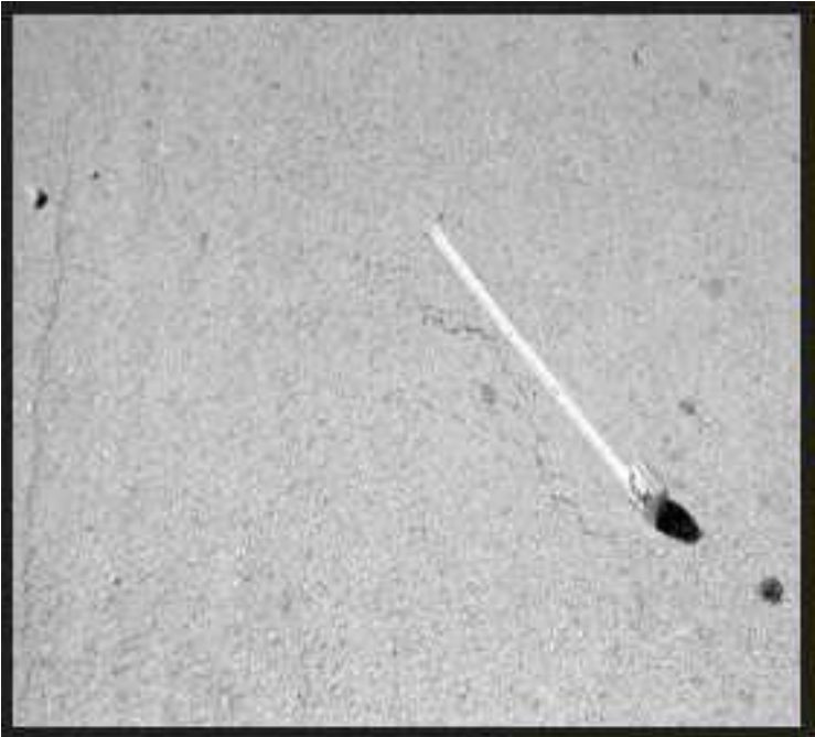
Figure A-65 Medium-Severity Slippage Cracking
