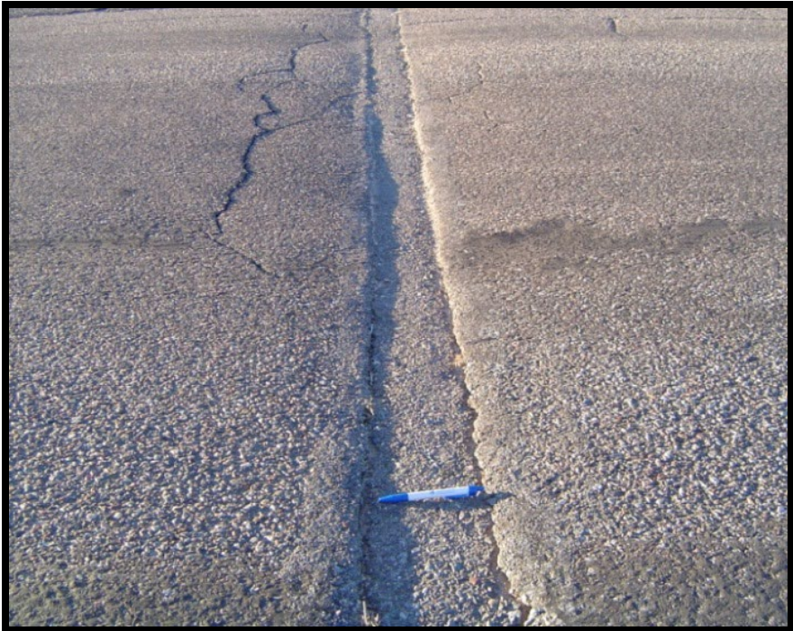
Figure A-190 High-Severity Patching
