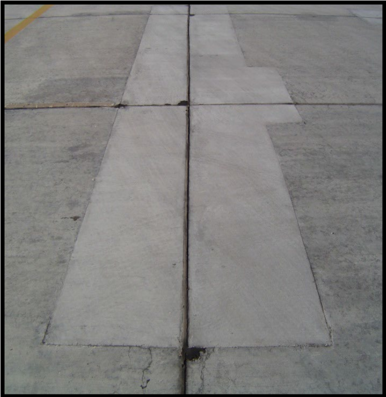
Figure A-251 Medium-Severity Large Patch
