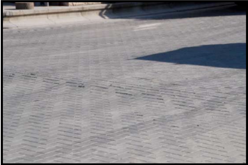
Figure A-321 Medium-Severity Heave
