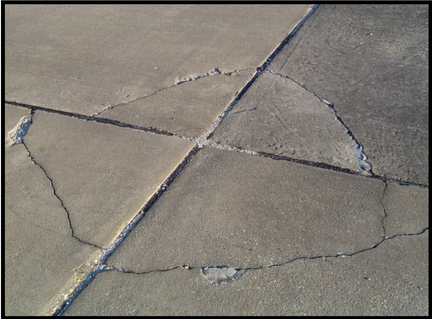
Figure A-231 High-Severity Corner Break
