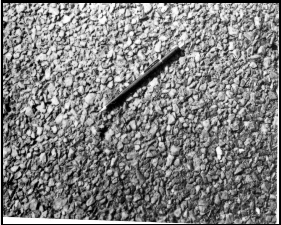
Figure A-201 Medium-Severity Raveling (PFC)
