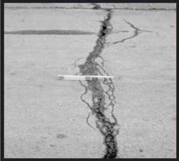
Figure A-32 High-Severity Joint Reflection Cracking
