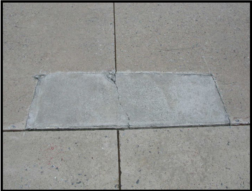
Figure A-248 High-Severity Small Patch
