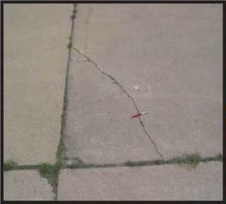
Figure A-83 Medium-Severity Corner Break
