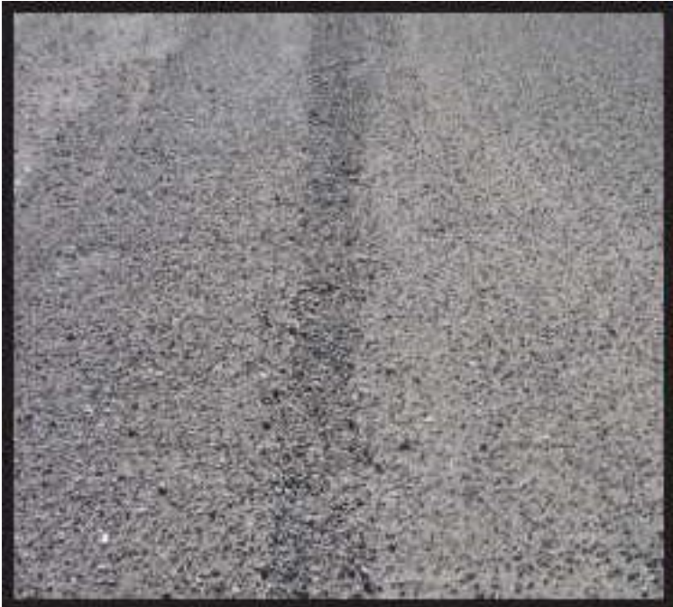
Figure A-71 High-Severity Raveling
