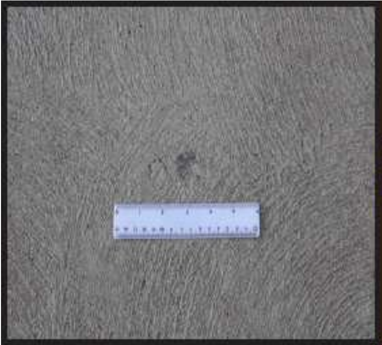
Figure A-134 Medium-Severity Scaling
