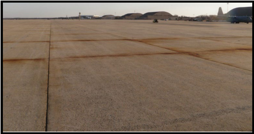
Figure A-257 Pumping Stains
