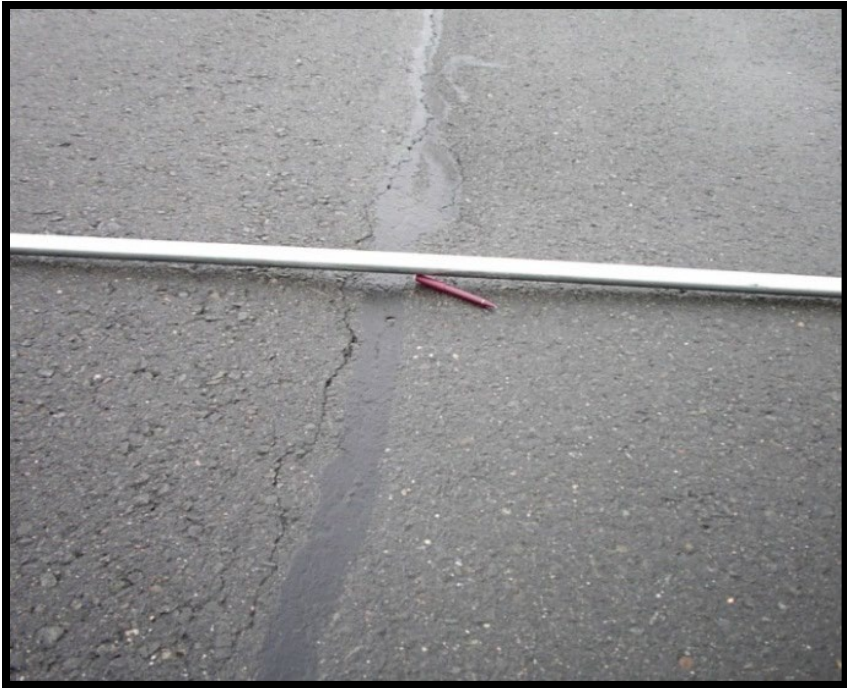
Figure A-168 Medium-Severity Depression
