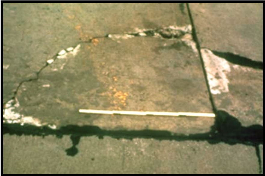
Figure A-231 High-Severity Corner Break
