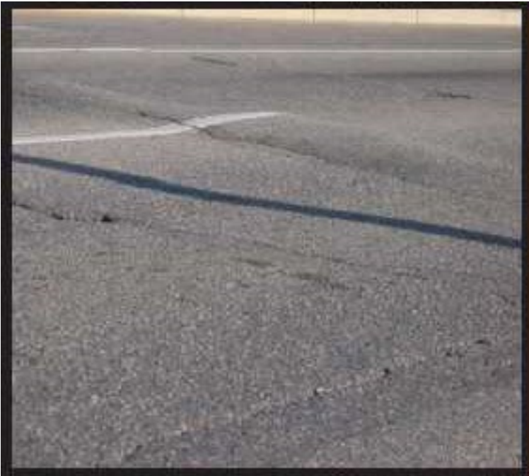
Figure A-14 Medium-Severity Bump or Sag
