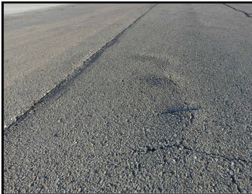
Figure A-215 Low-Severity Swell
