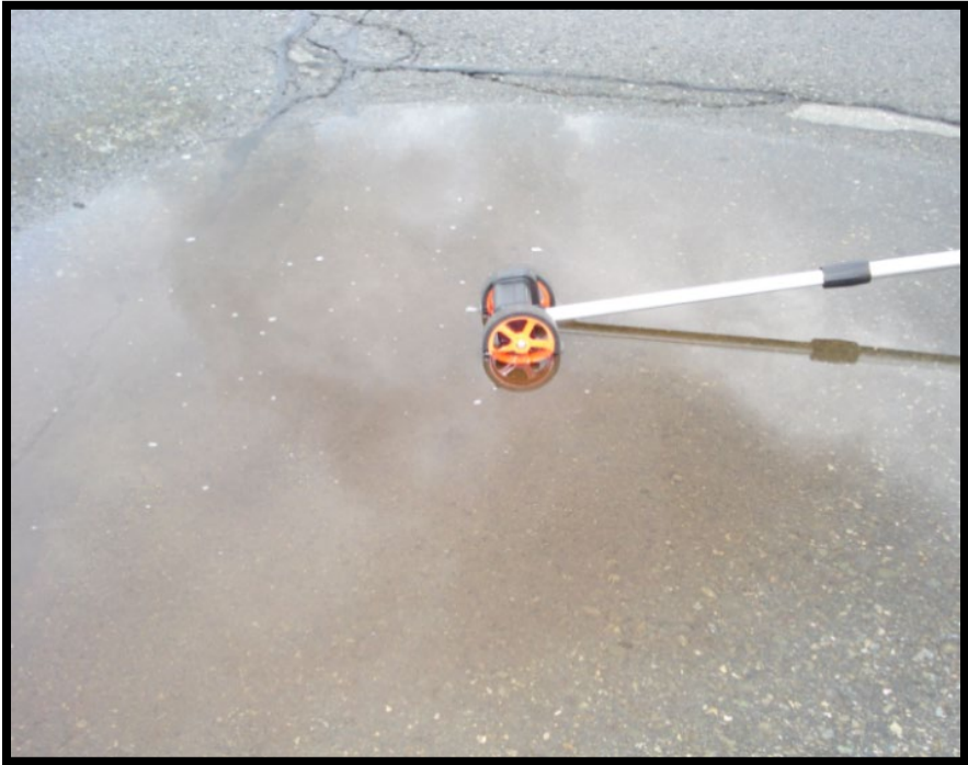
Figure A-170 High-Severity Depression
