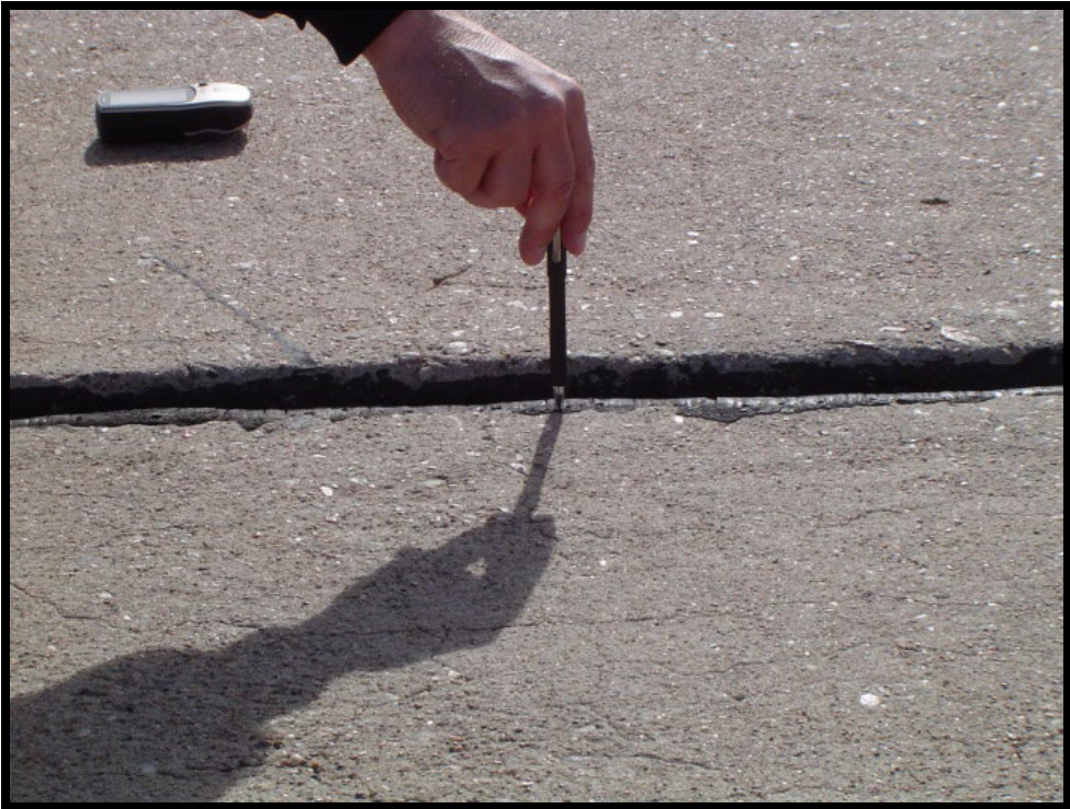
Figure A-265 High-Severity Settlement or Faulting
