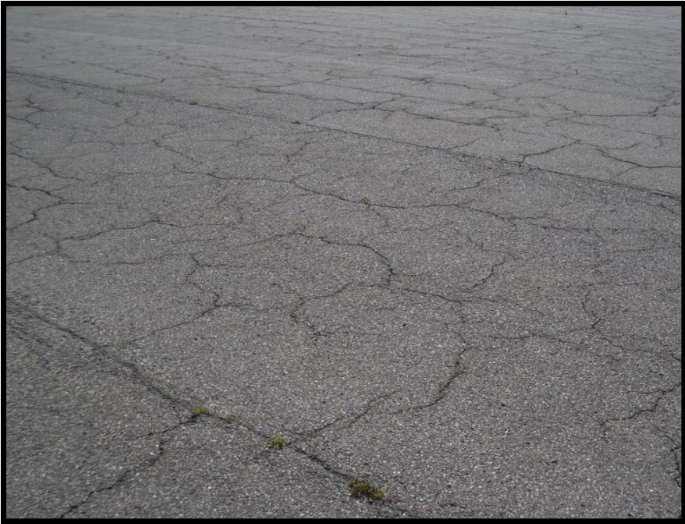
Figure A-160 High-Severity Block Cracking
