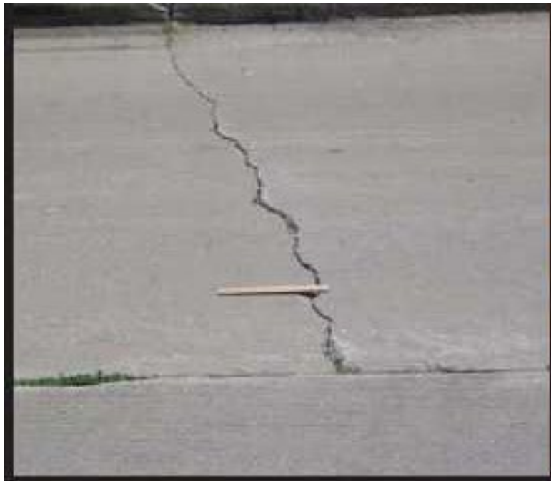
Figure A-107 Medium-Severity Linear Cracking
