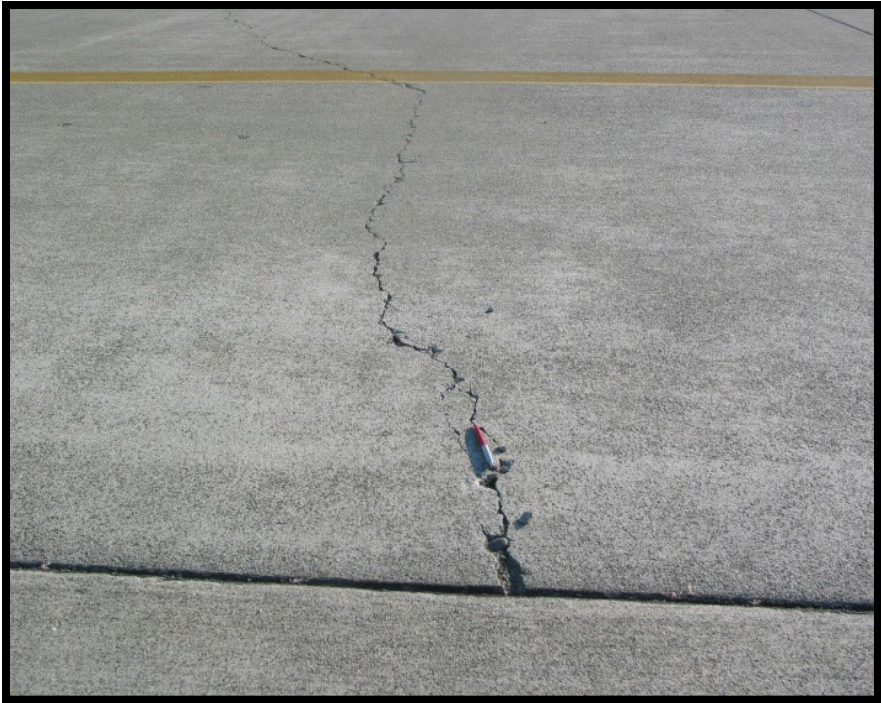
Figure A-235 High-Severity Linear Cracking
