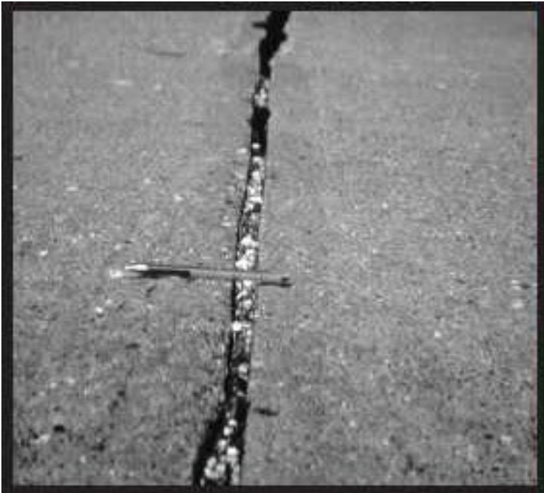
Figure A-100 High-Severity Joint Seal Damage
