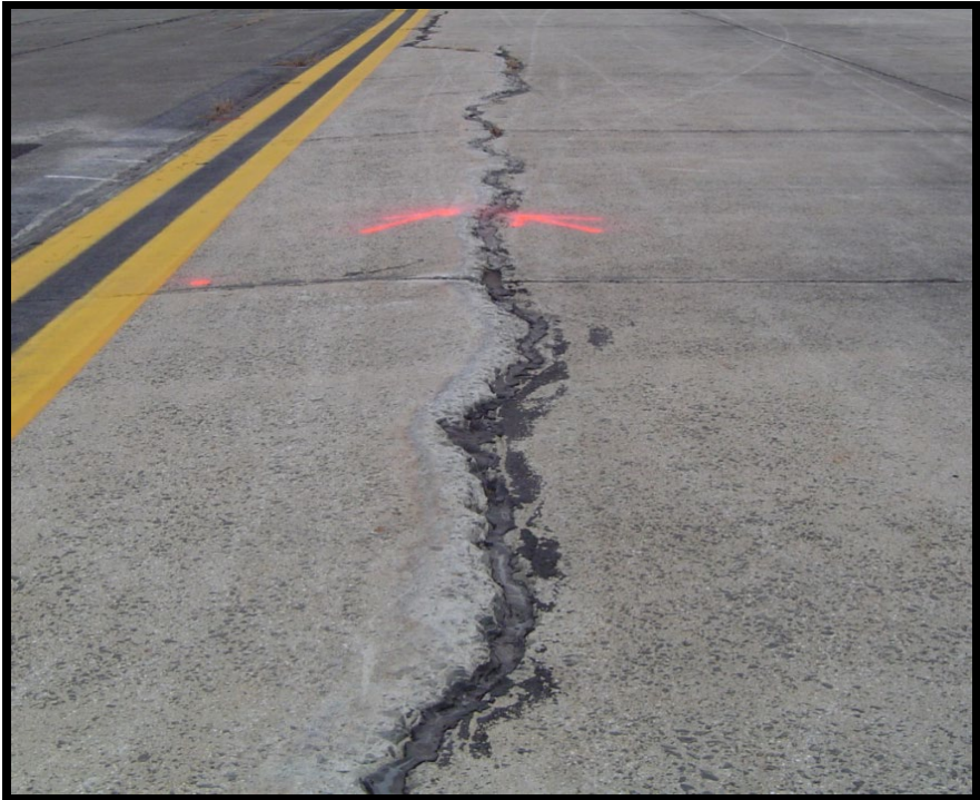
Figure A-225 Low-Severity Blowup
