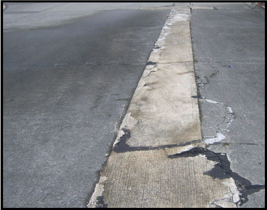
Figure A-225 Low-Severity Blowup
