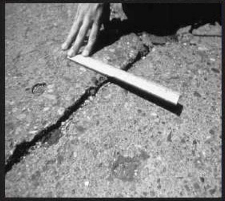
Figure A-96 High-Severity Faulting
