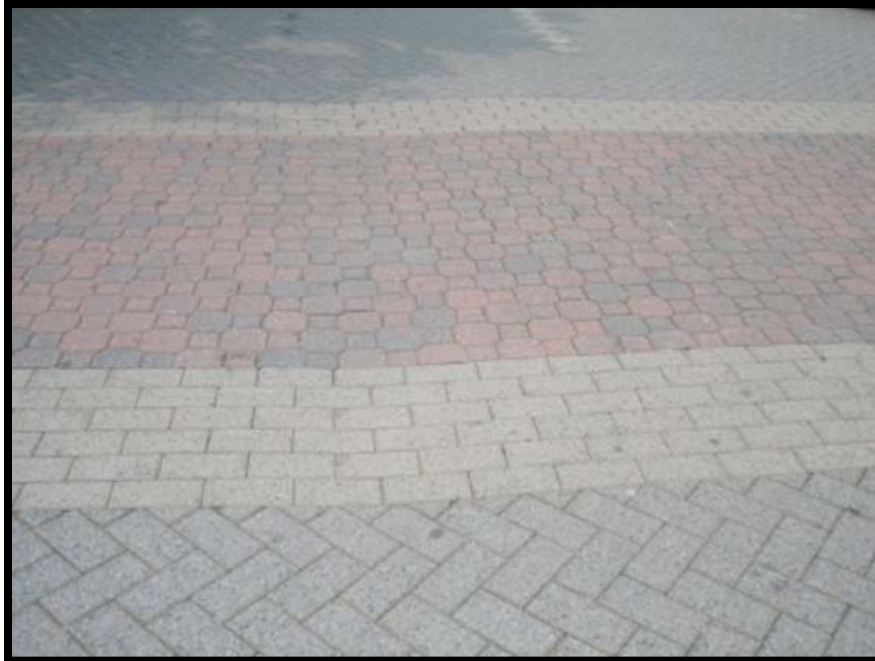
Figure A-305 Medium-Severity Depression
