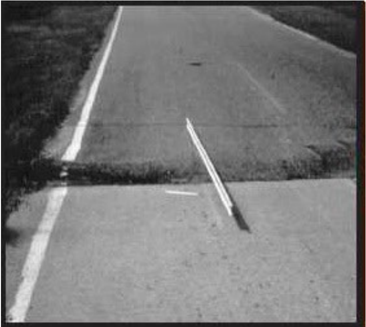
Figure A-62 High-Severity Shoving
