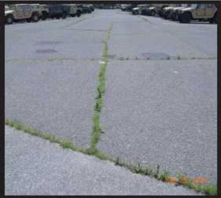
Figure A-32 High-Severity Joint Reflection Cracking
