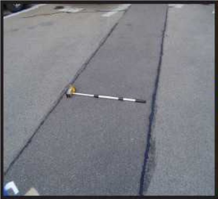
Figure A-43 Medium-Severity Patch and Utility Cut Patching
