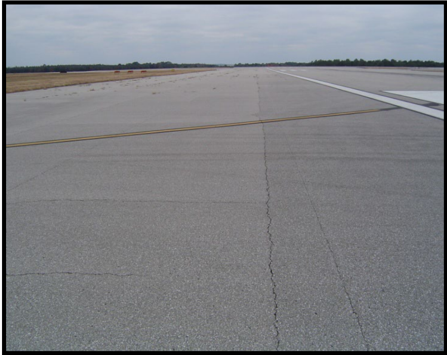
Figure A-175 Medium-Severity Joint Reflection Cracking
