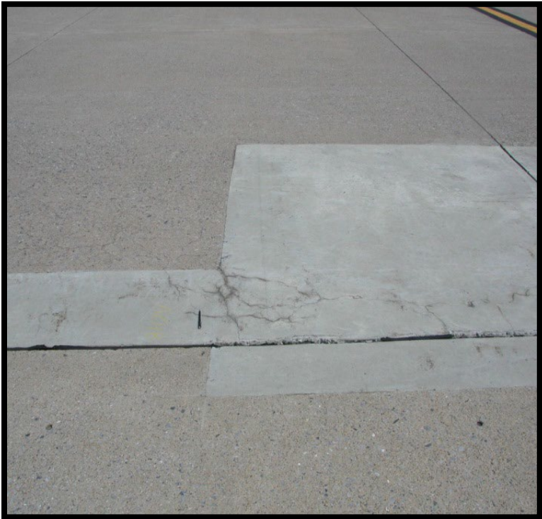
Figure A-251 Medium-Severity Large Patch
