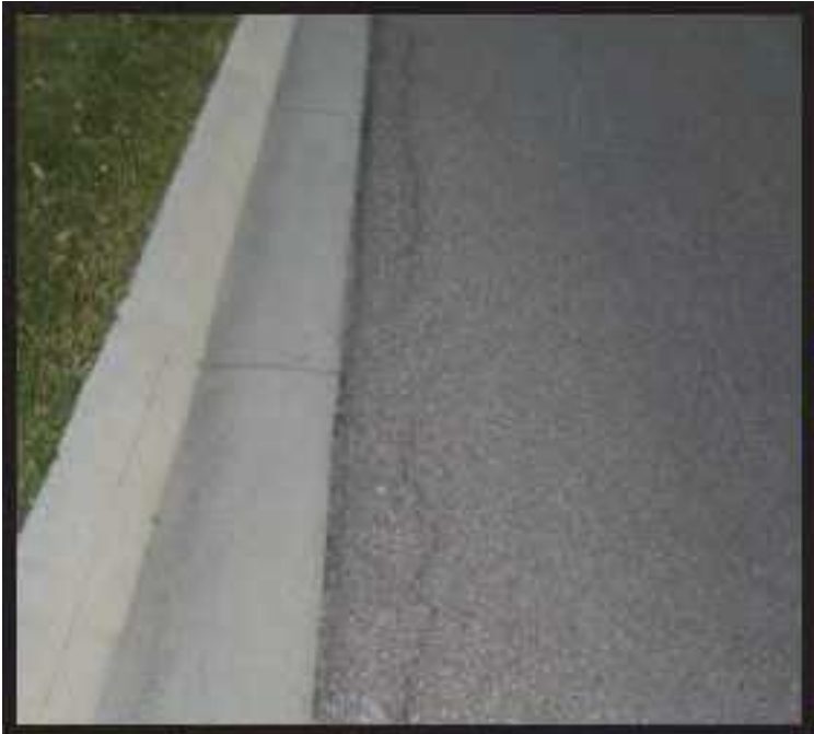
Figure A-27 Medium-Severity Edge Cracking
