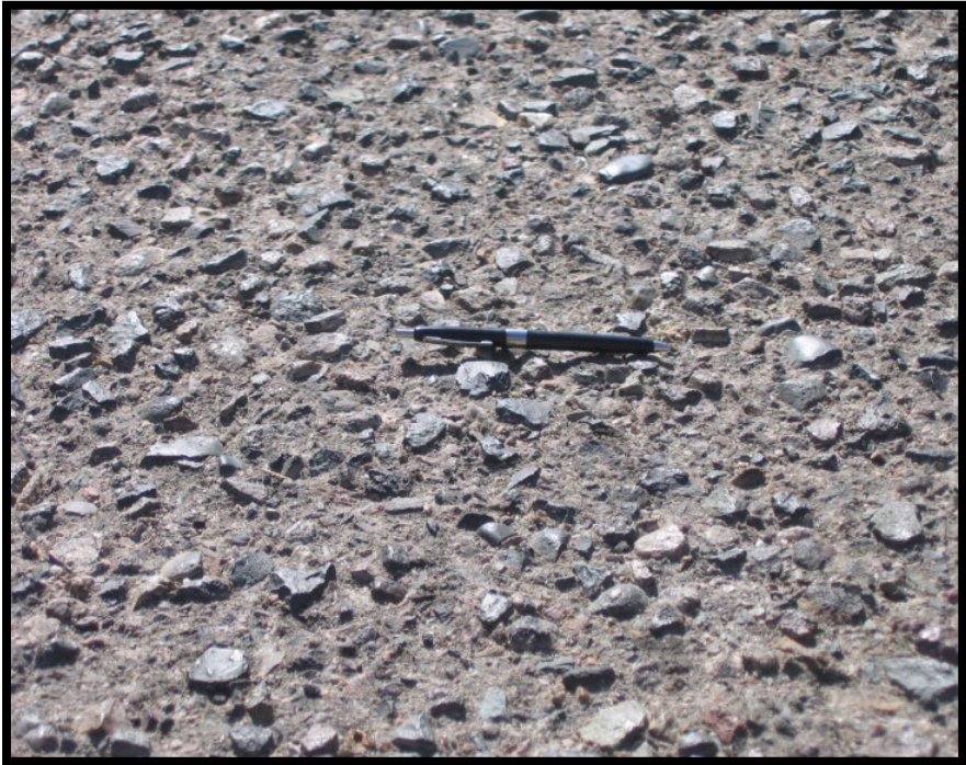
Figure A-221 High-Severity Weathering
