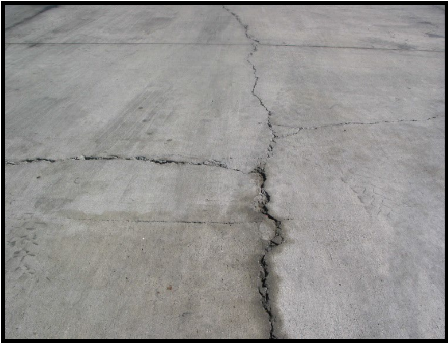
Figure A-269 High-Severity Shattered Slab/Intersecting Cracks
