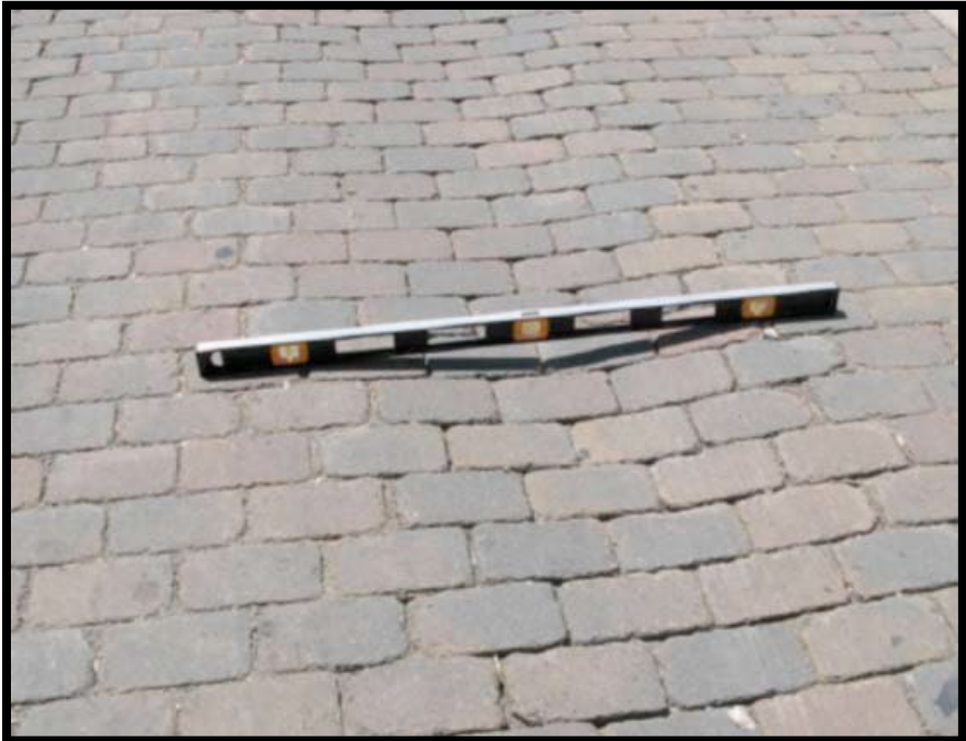
Figure A-342 High-Severity Rutting
