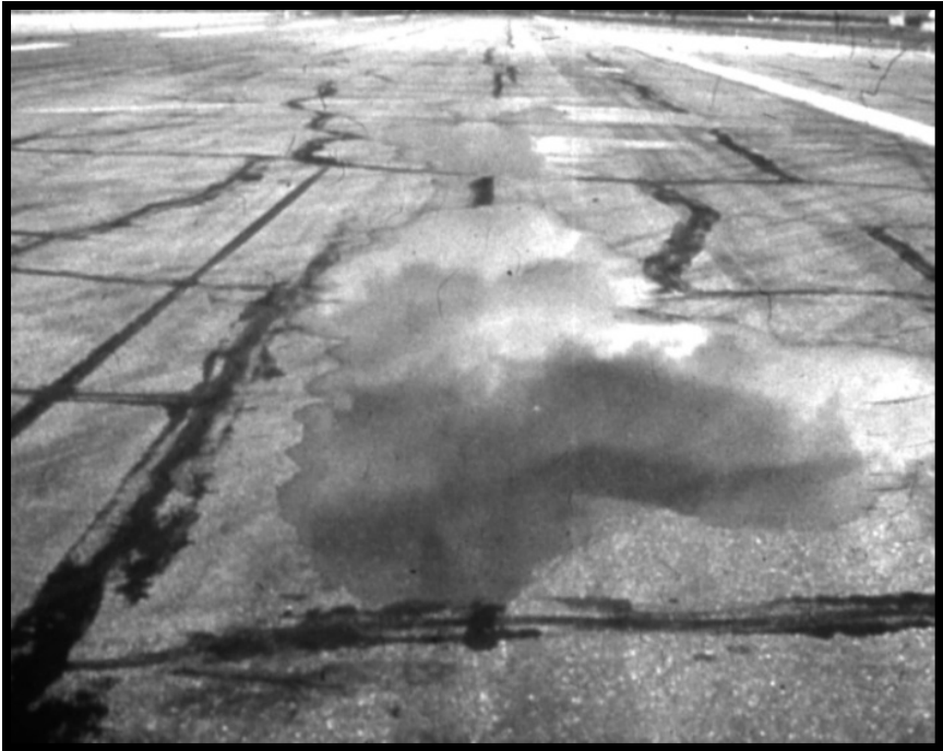
Figure A-170 High-Severity Depression
