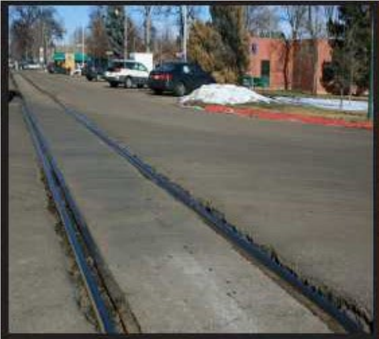
Figure A-54 High-Severity Railroad Crossing
