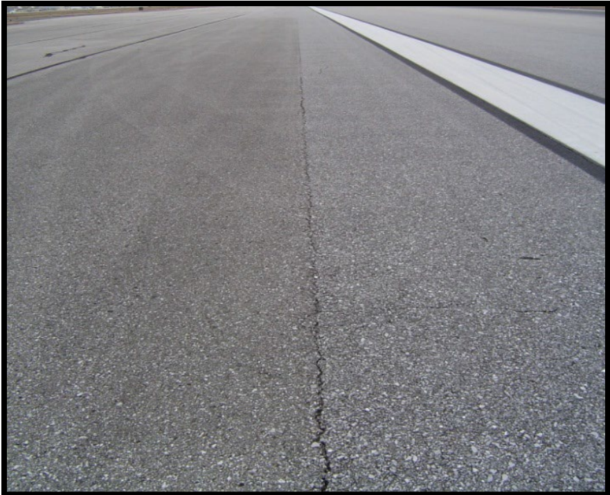
Figure A-179 Medium-Severity L&T Cracking
