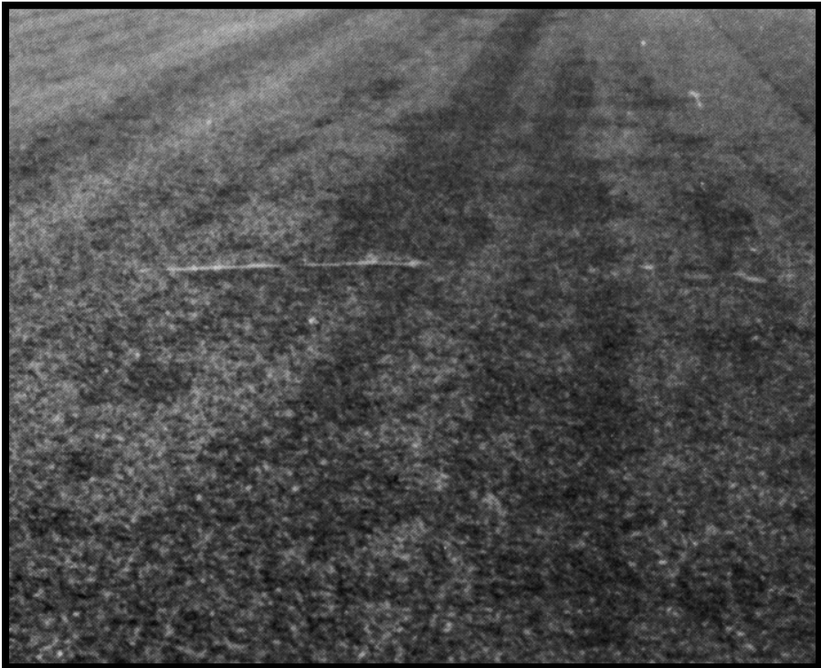
Figure A-201 Medium-Severity Raveling (PFC)
