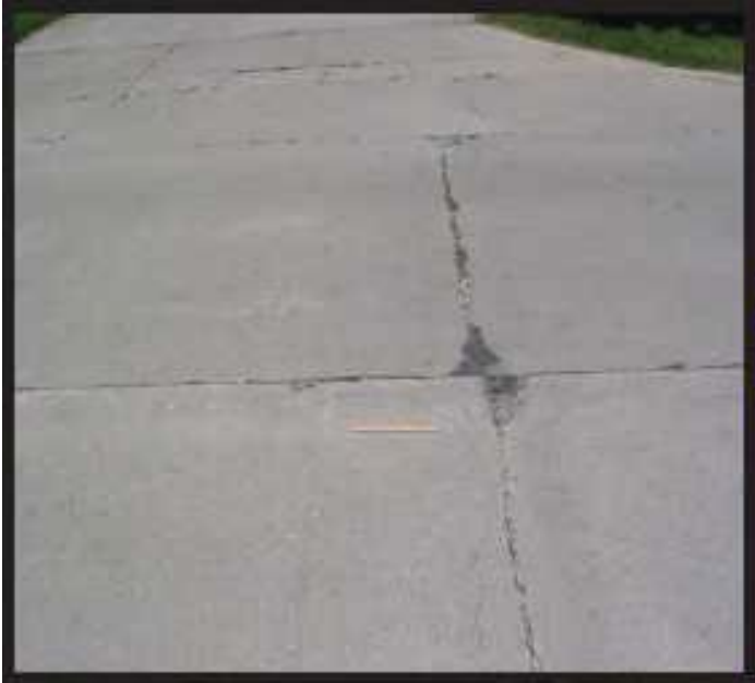
Figure A-91 Medium-Severity Durability Cracking
