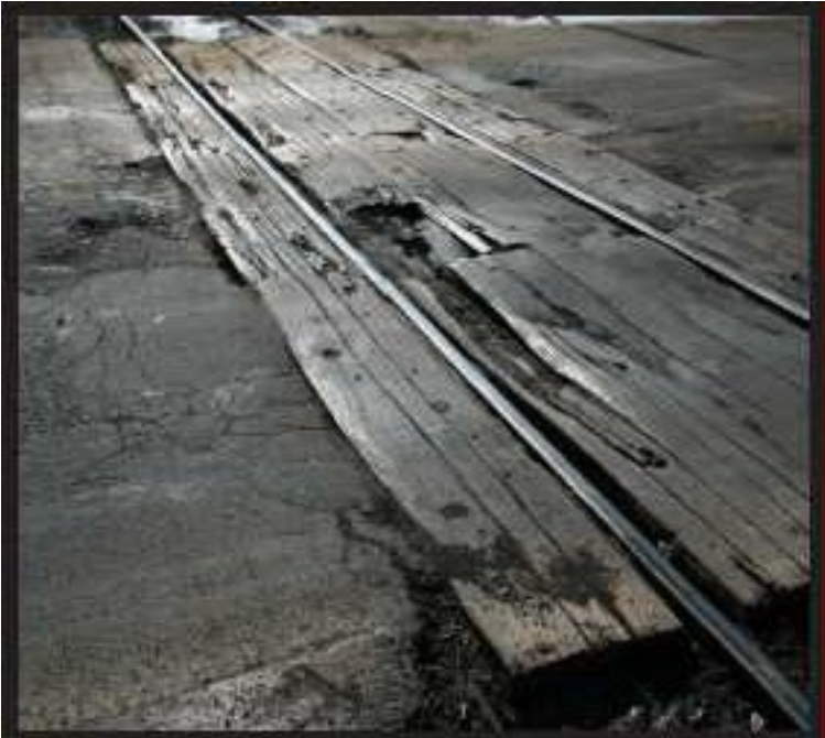
Figure A-54 High-Severity Railroad Crossing
