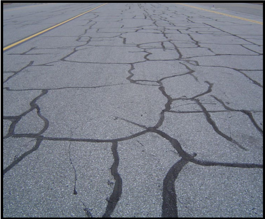
Figure A-156 Low-Severity Block Cracking
