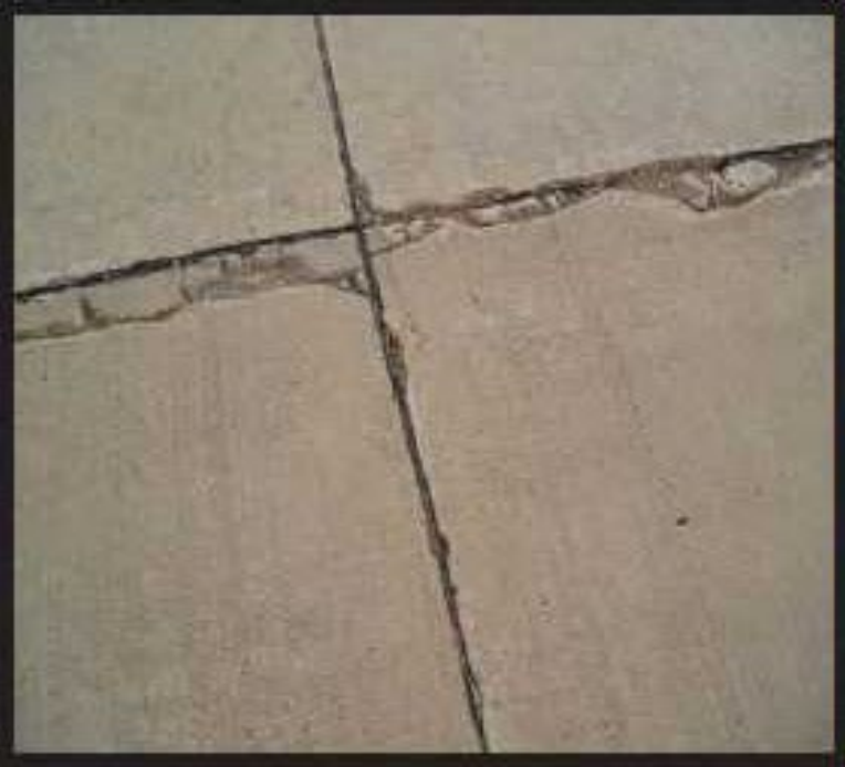
Figure A-144 Medium-Severity Joint Spall
