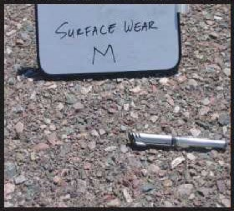
Figure A-75 High-Severity Weathering
