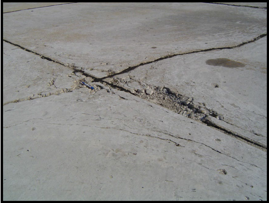
Figure A-240 High-Severity "D" Cracking
