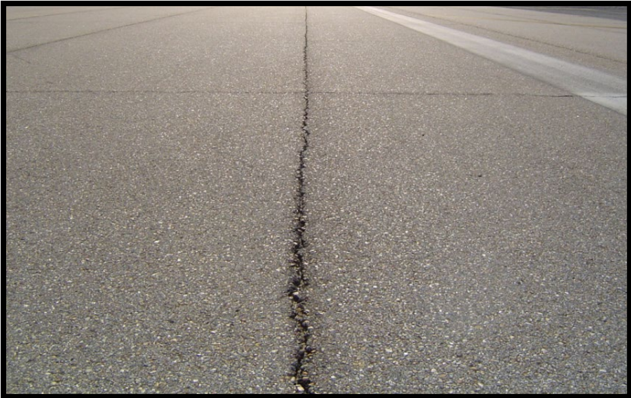
Figure A-175 Medium-Severity Joint Reflection Cracking
