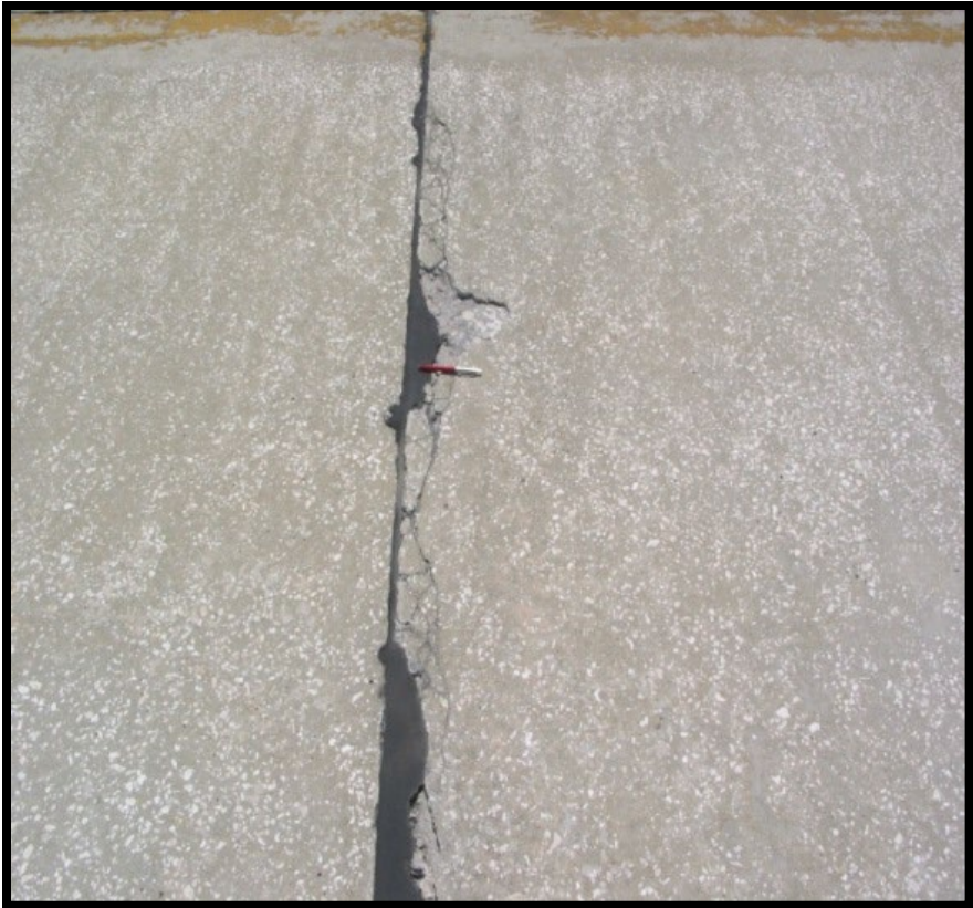
Figure A-276 High-Severity Joint Spall
