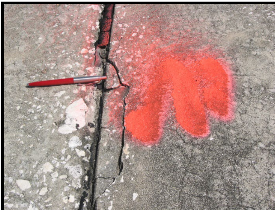
Figure A-274 Medium-Severity Joint Spall
