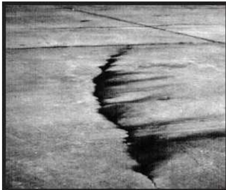
Figure A-122 Pumping
