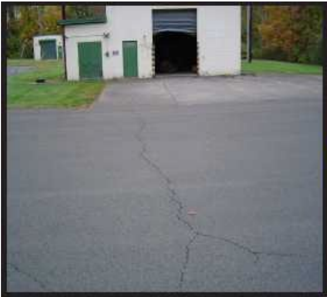
Figure A-39 Medium-Severity Longitudinal and Transverse Cracking
