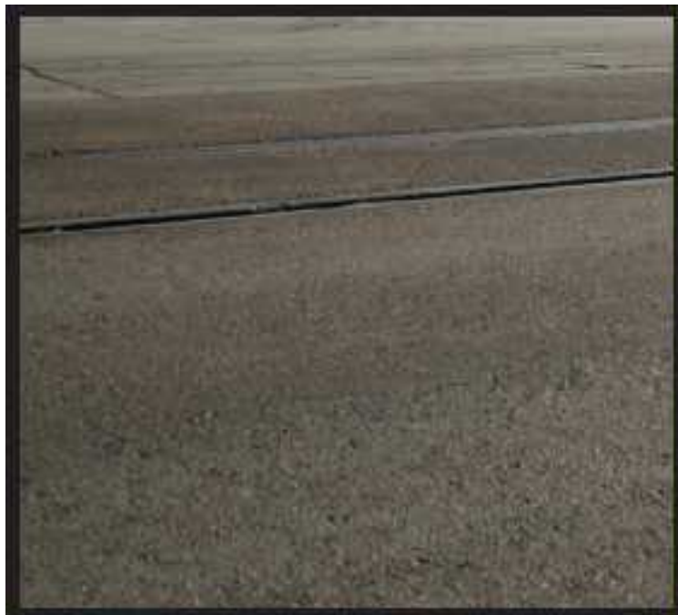
Figure A-52 Low-Severity Railroad Crossing
