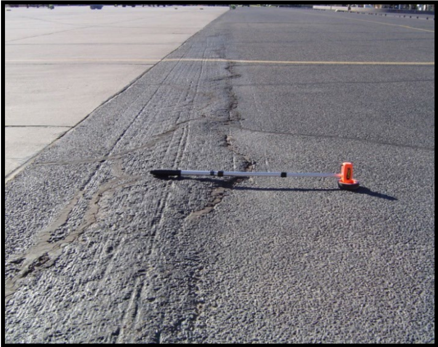
Figure A-210 Medium-Severity Shoving
