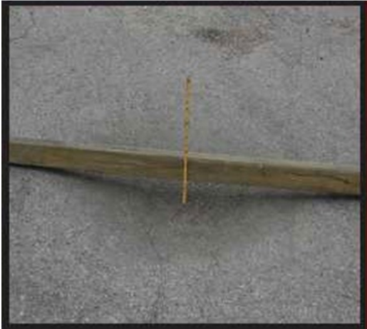
Figure A-24 High-Severity Depression
