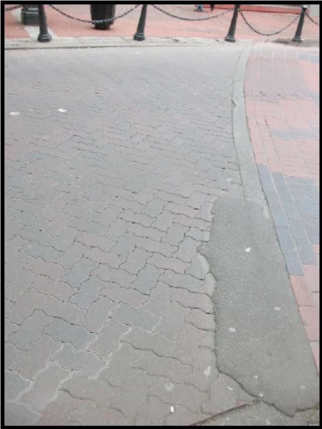
Figure A-337 Medium-Severity Patch
