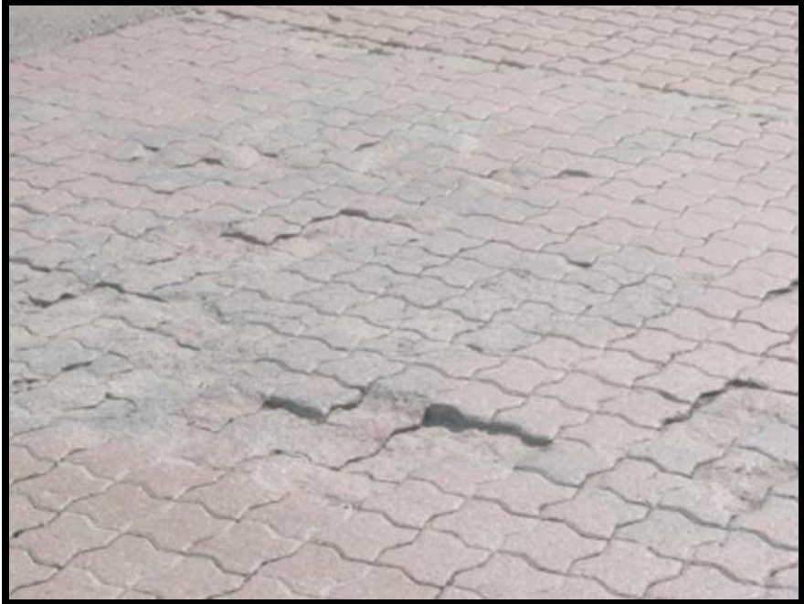
Figure A-302 High-Severity Damaged Pavers
