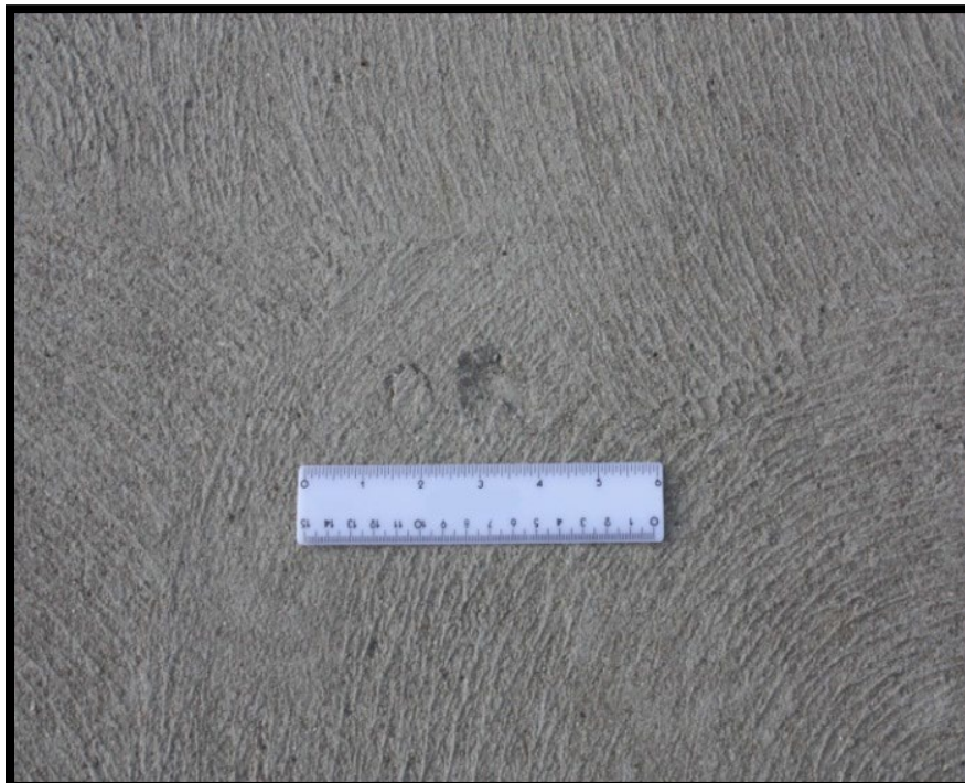
Figure A-259 Low-Severity Scaling
