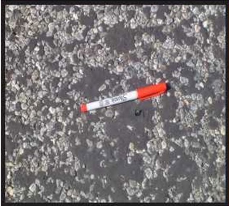
Figure A-7 High-Severity Bleeding
