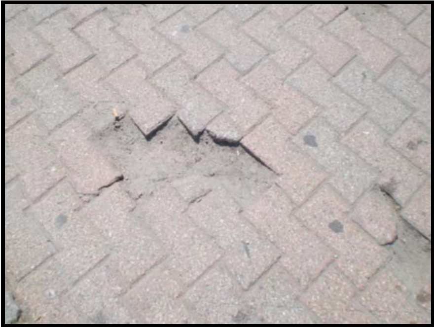
Figure A-334 High-Severity Missing Pavers
