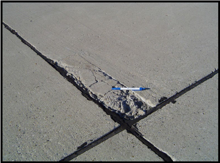
Figure A-248 High-Severity Small Patch
