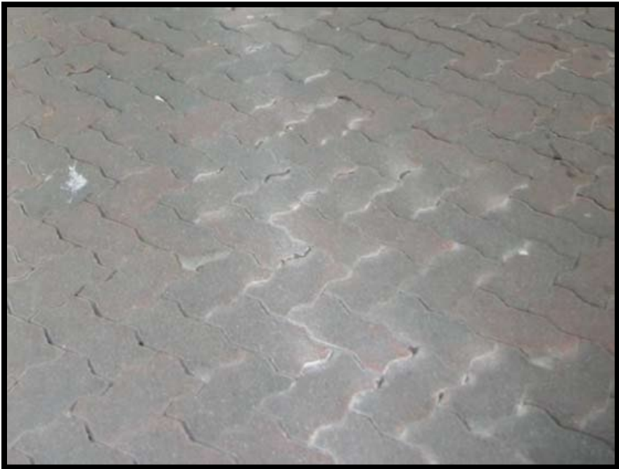
Figure A-329 Medium-Severity Joint Sand Loss
