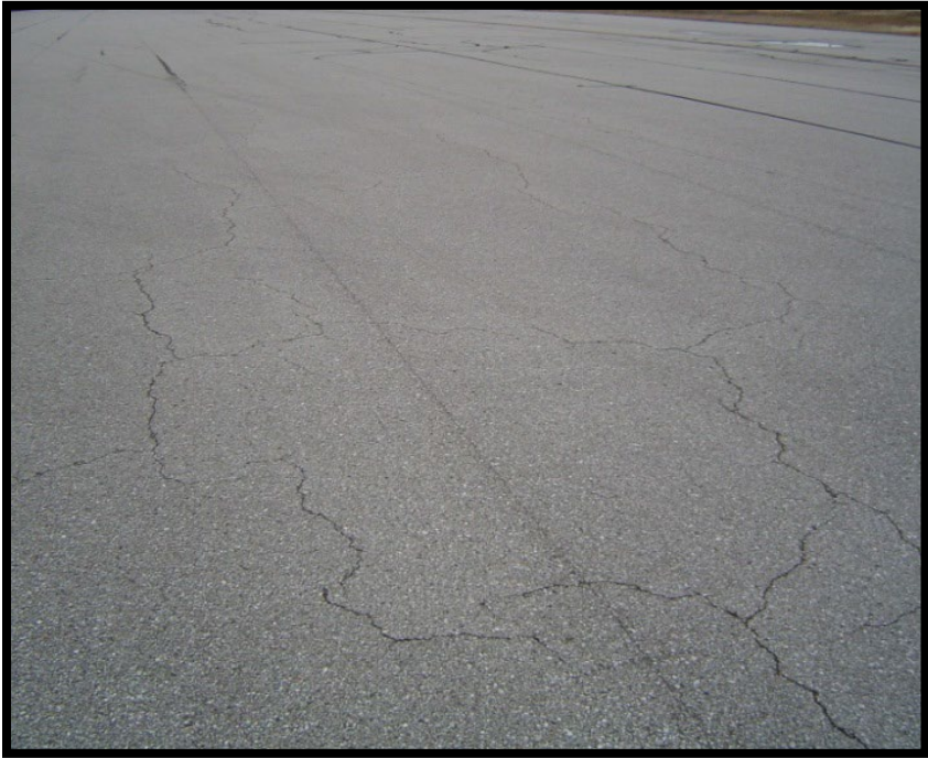
Figure A-156 Low-Severity Block Cracking
