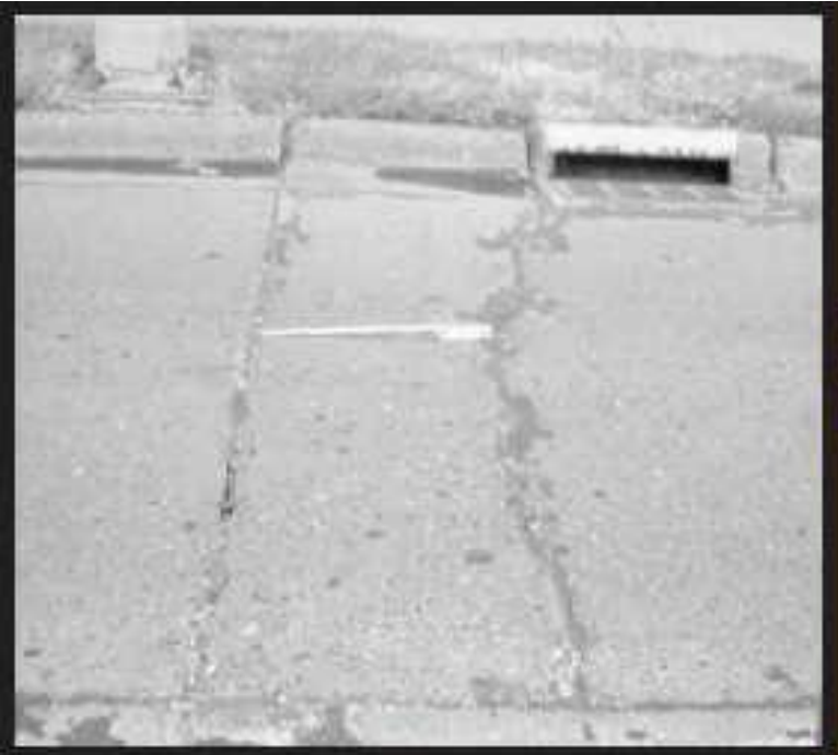
Figure A-126 Medium-Severity Punchout
