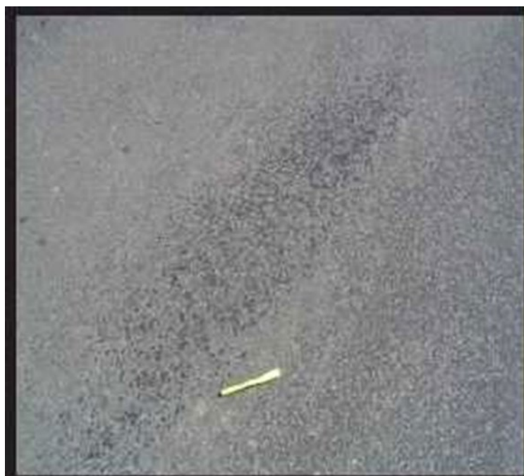
Figure A-5 Low-Severity Bleeding
