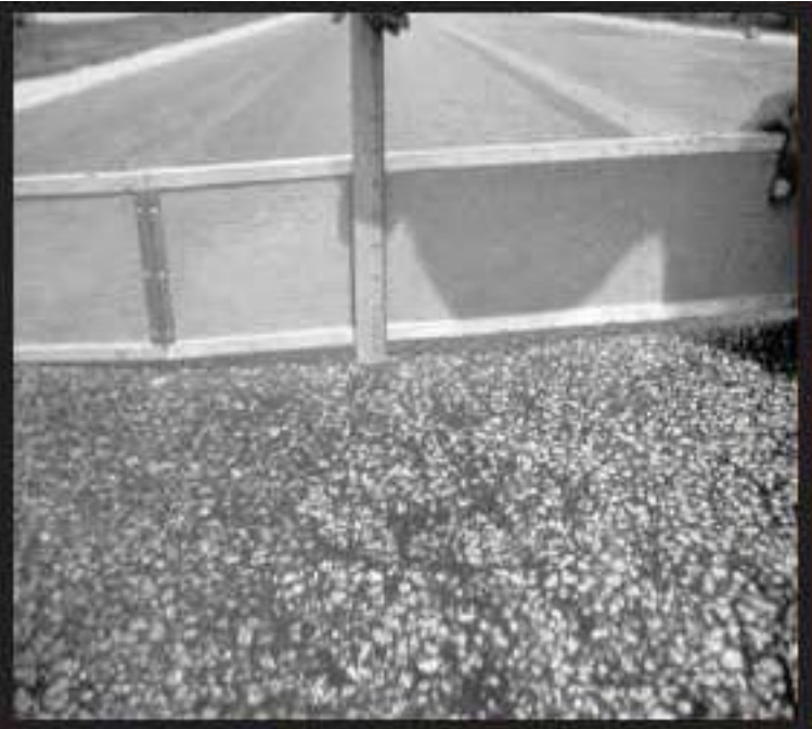
Figure A-57 Medium-Severity Rutting
