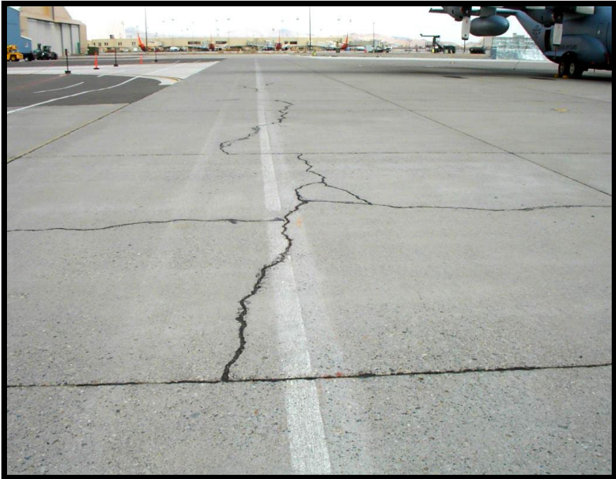
Figure A-269 High-Severity Shattered Slab/Intersecting Cracks
