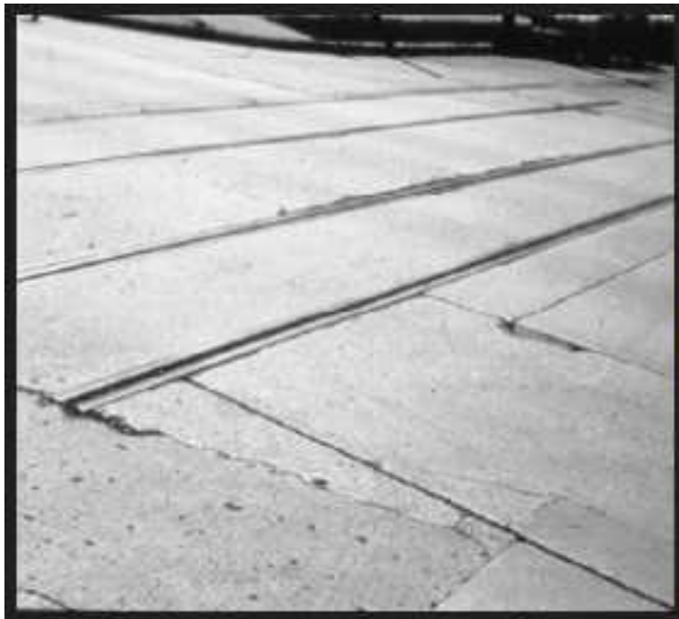
Figure A-129 Low-Severity Railroad Crossing
