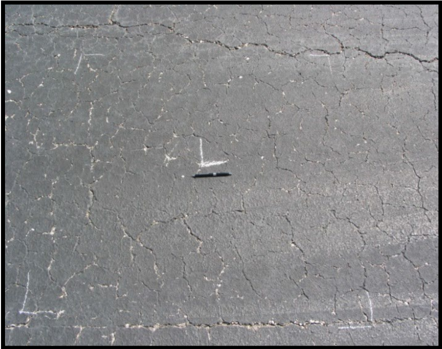
Figure A-198 Medium-Severity Raveling (Slurry Seal/Coal Tar Over Dense Mix)
