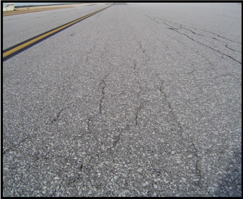
Figure A-149 Medium-Severity Alligator Cracking
