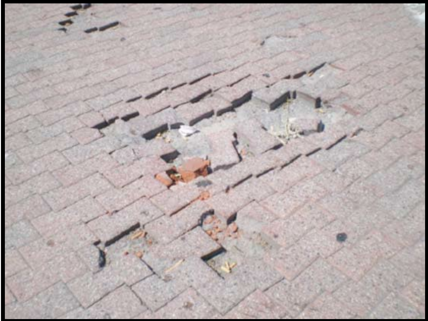
Figure A-334 High-Severity Missing Pavers
