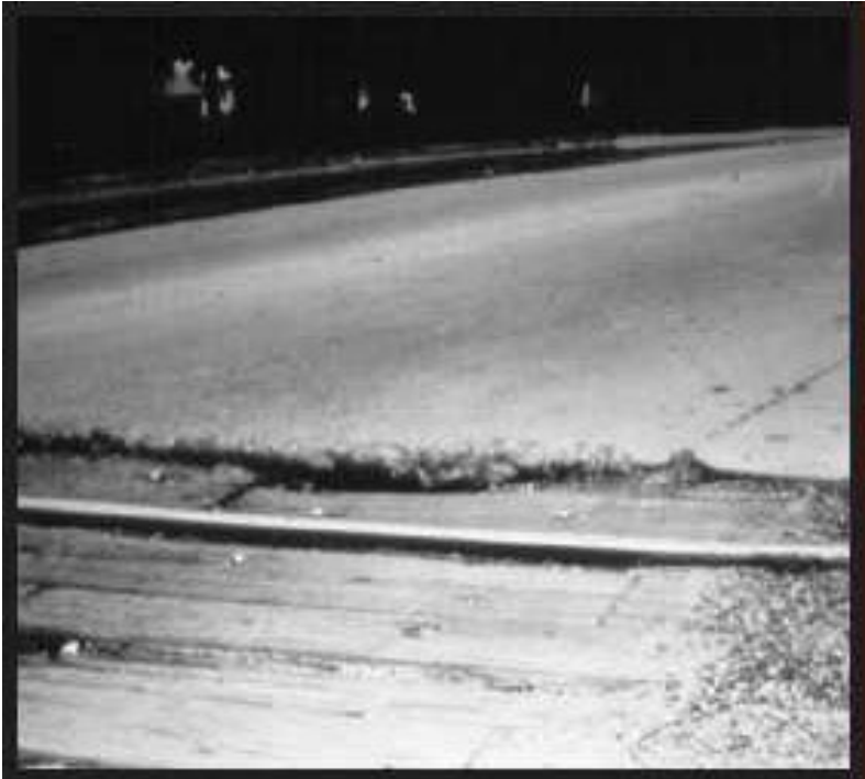
Figure A-131 High-Severity Railroad Crossing
