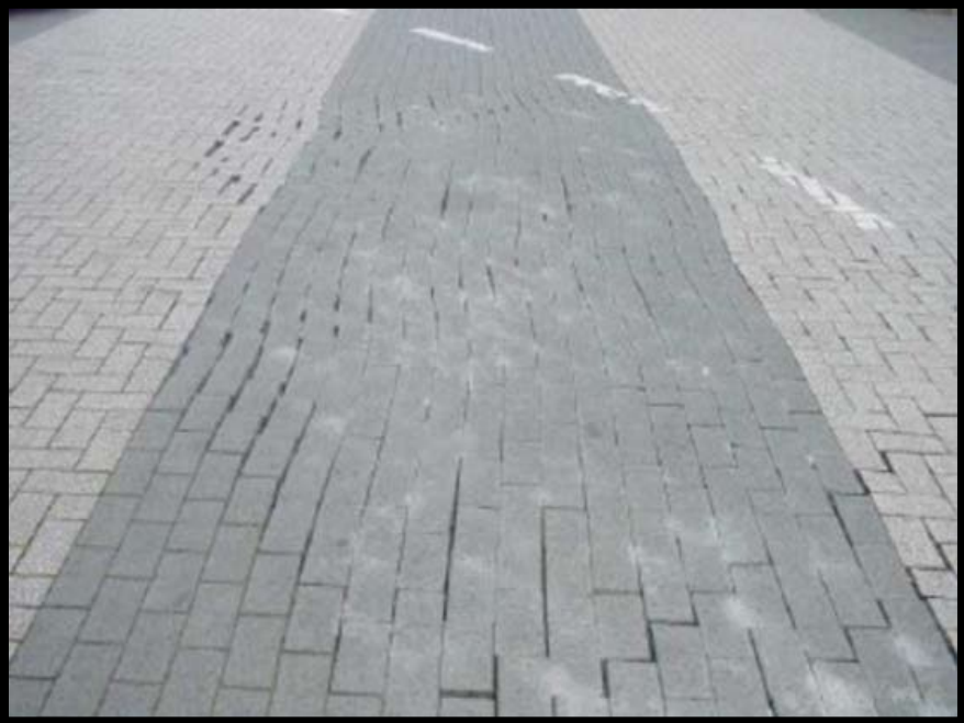
Figure A-310 High-Severity Edge Restraint Damage
