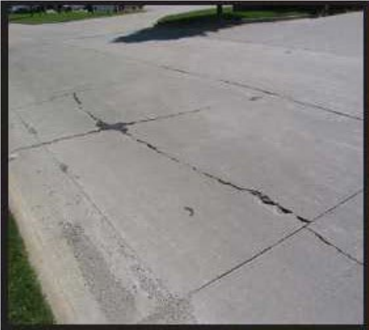
Figure A-88 High-Severity Divided Slab
