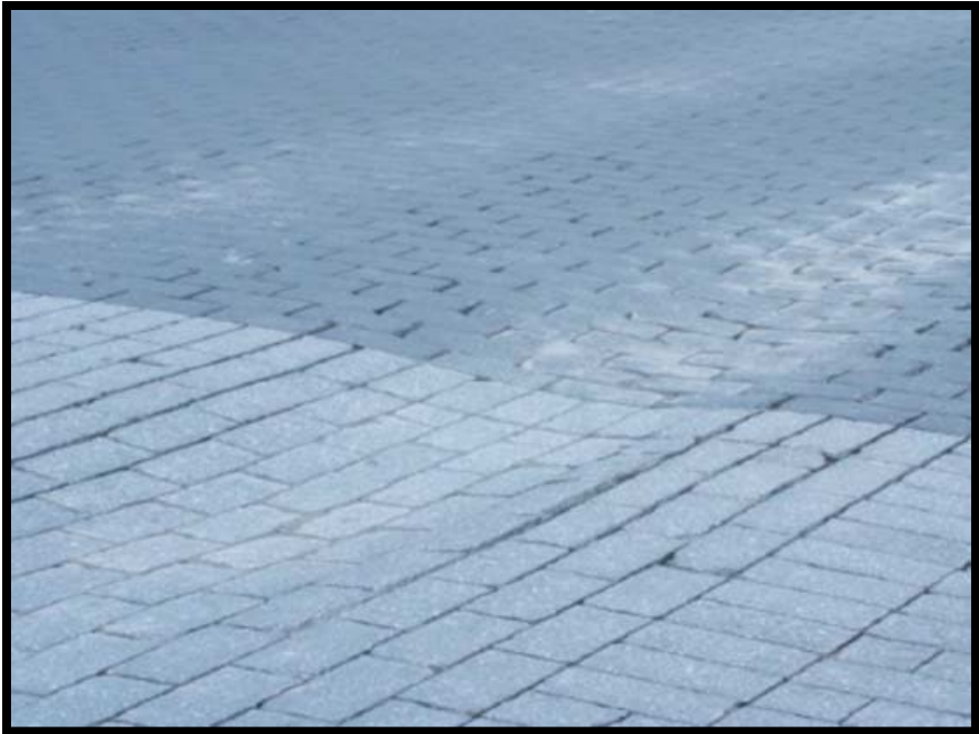
Figure A-342 High-Severity Rutting
