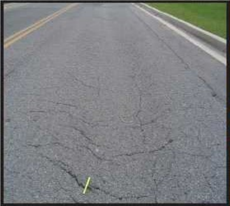
Figure A-65 Medium-Severity Slippage Cracking
