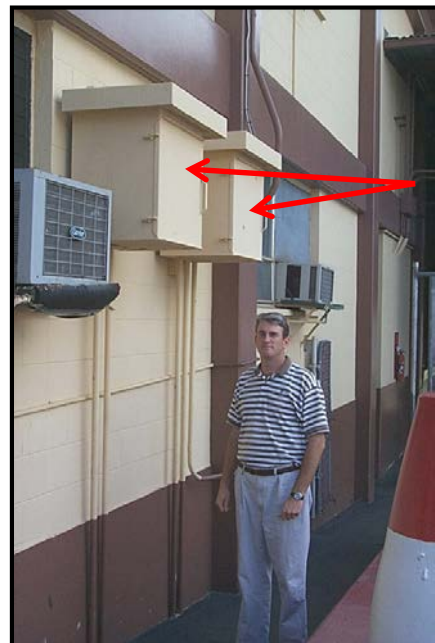
Figure B-12 Rectifiers Located for Ease of Maintenance. .
