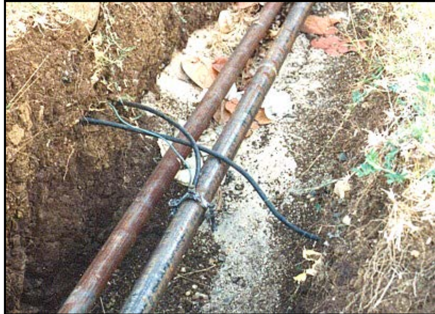
Figure 4-5 Mechanical Connection of Wiring to the Structure
