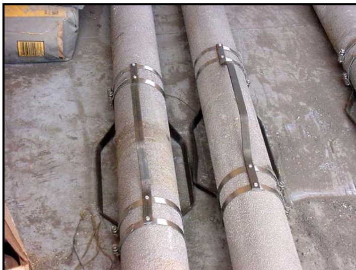
Figure B-22 Centralizers Installed on High Silicon Cast Iron Anodes
