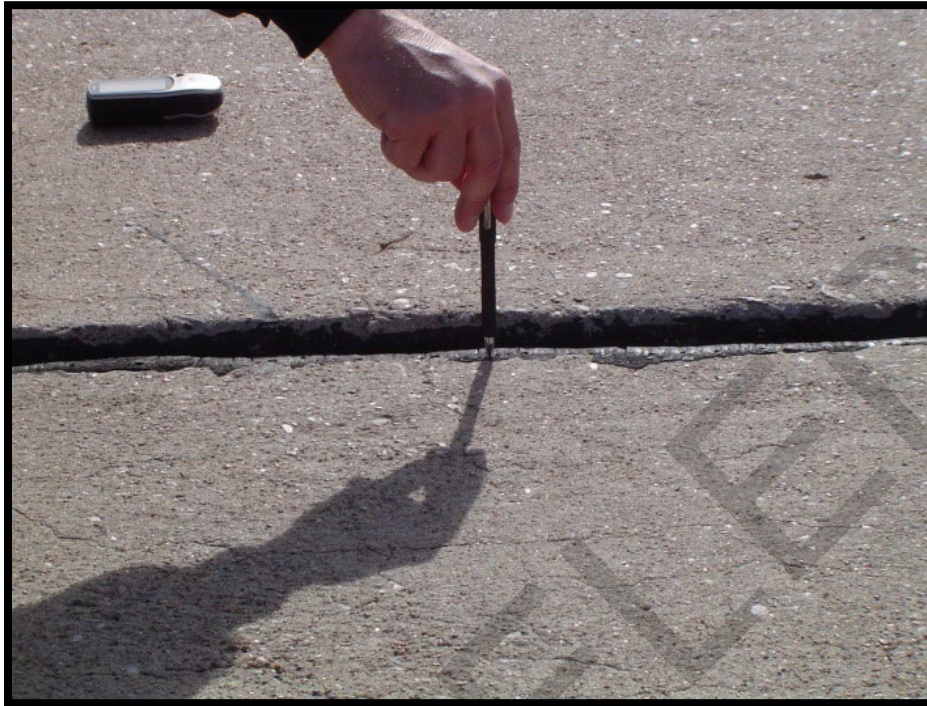
Figure B-32 High-Severity Settlement or Faulting
