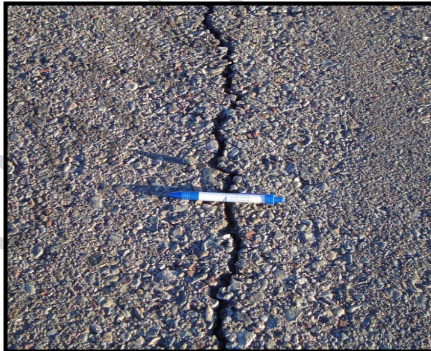
Figure A-25 Medium-Severity L&T Cracking
