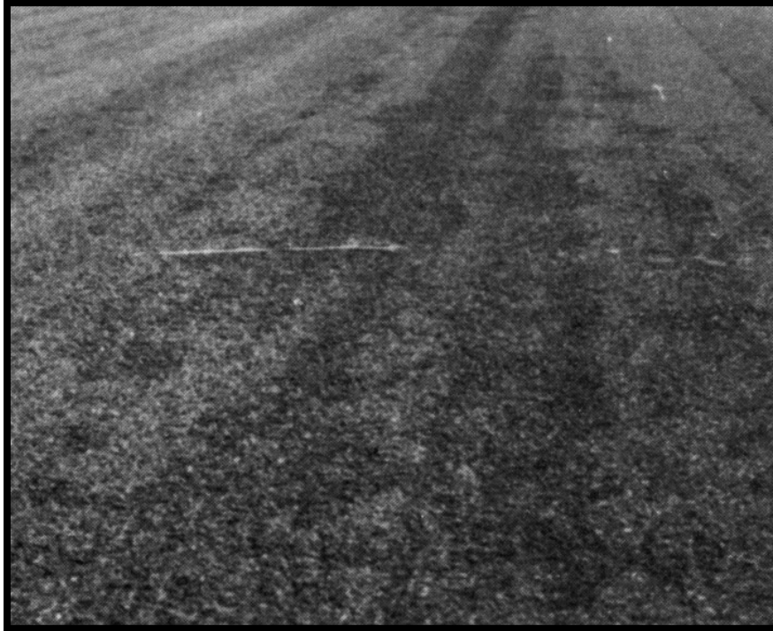
Figure A-44 Medium-Severity Raveling (PFC)
