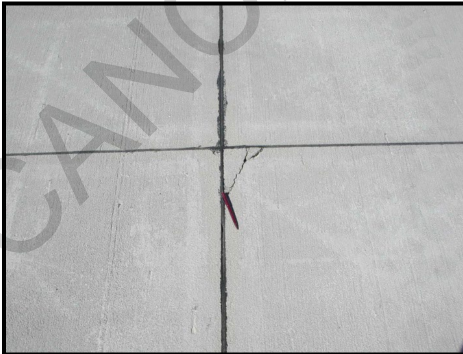
Figure B-42 Medium-Severity Corner Spall
