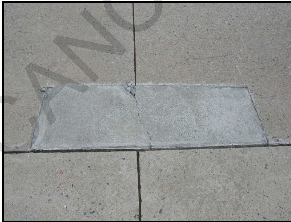
Figure B-19 Medium-Severity Small Patch
