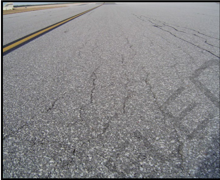
Figure A-2 Medium-Severity Alligator Cracking
