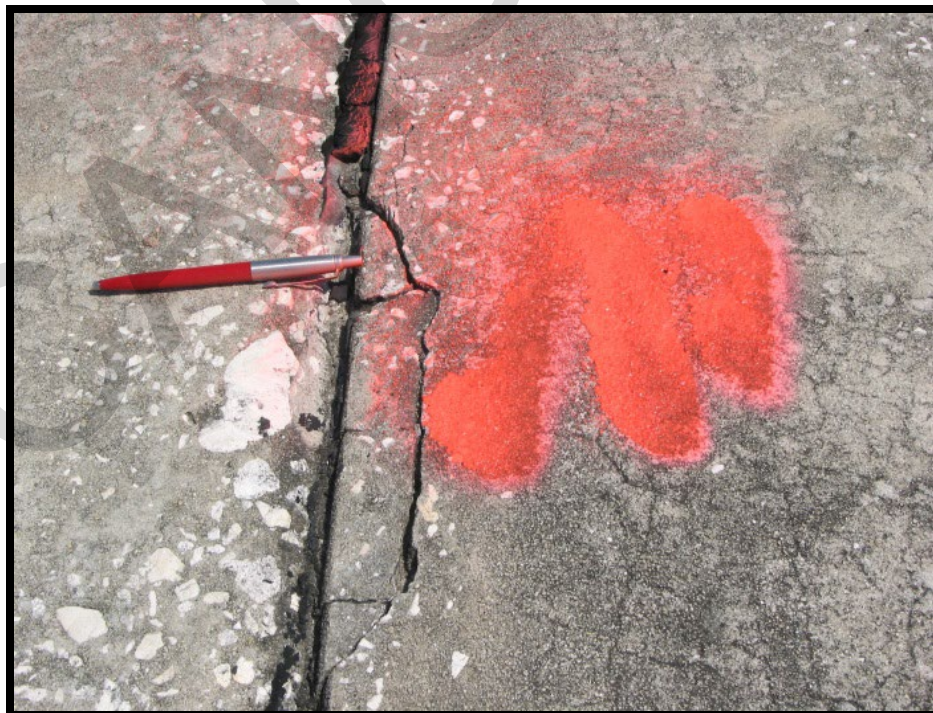
Figure B-38 Medium-Severity Joint Spall
