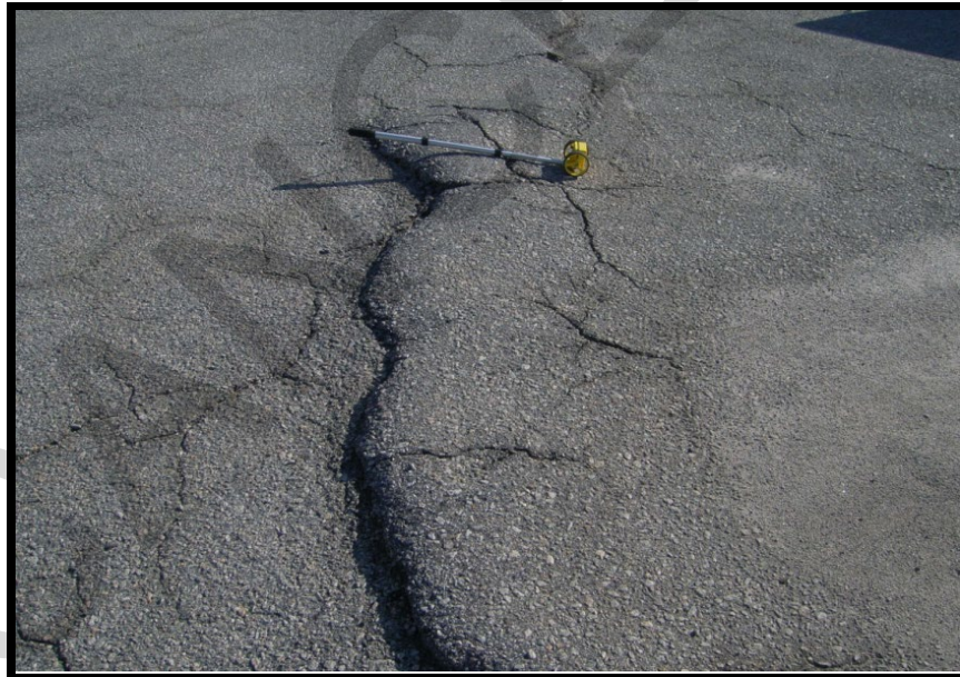
Figure A-53 High-Severity Swell
