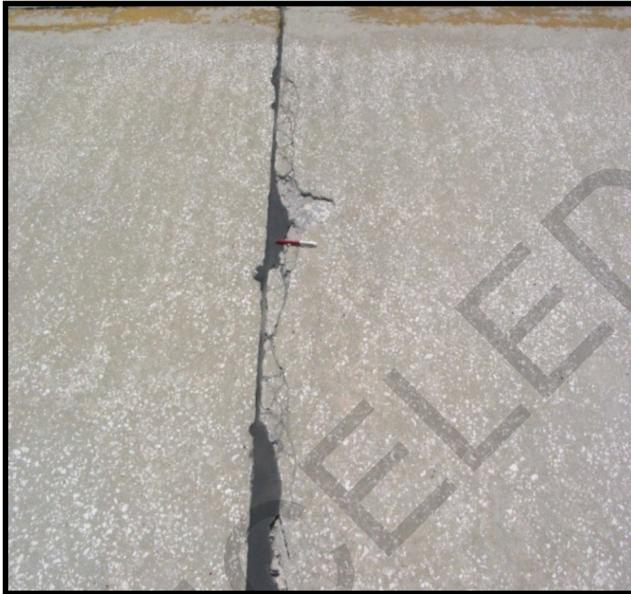
Figure B-40 High-Severity Joint Spall
