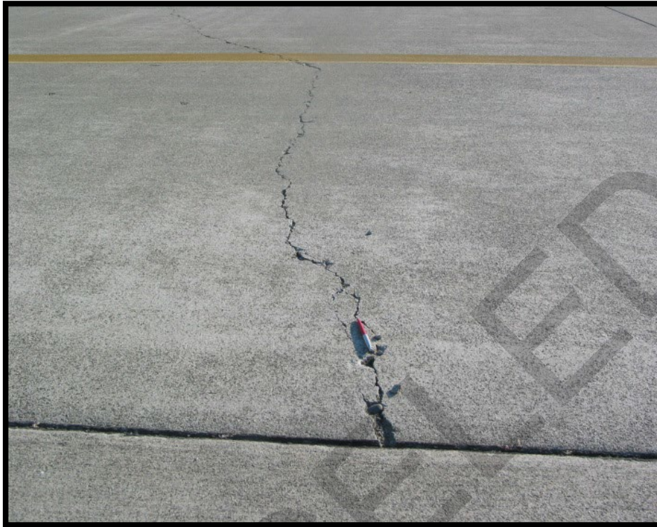
Figure B-10 High-Severity Linear Cracks
