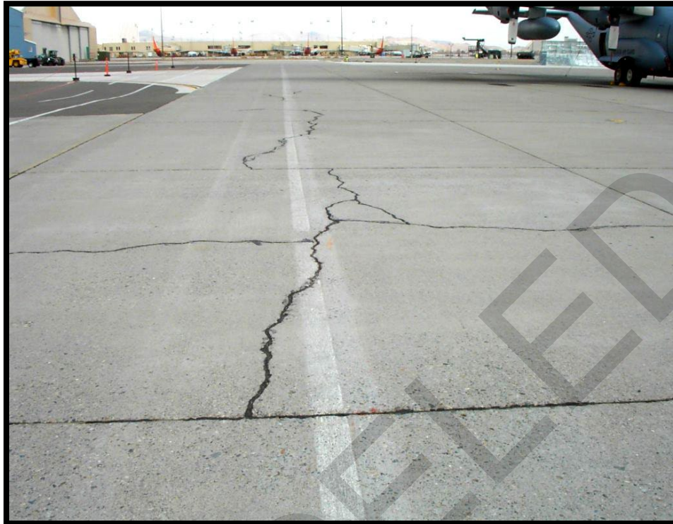
Figure B-35 High-Severity Shattered Slab/Intersecting Cracks
