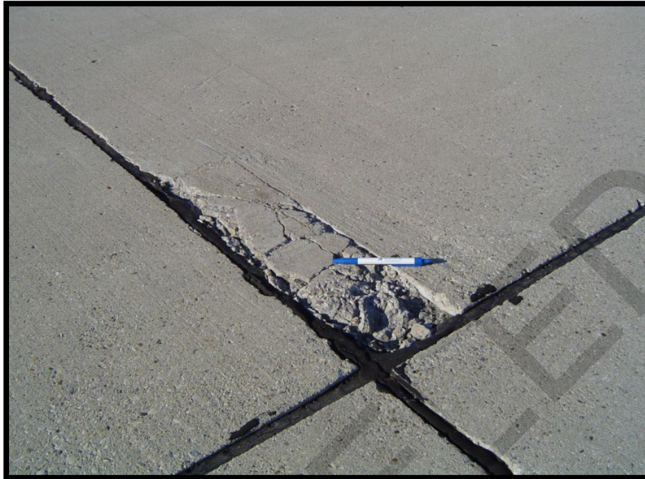
Figure B-20 High-Severity Small Patch
