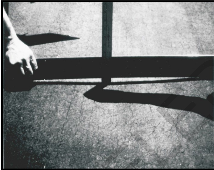
Figure A-18 High-Severity Depression
