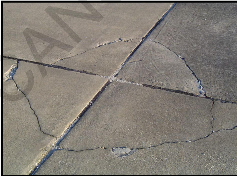
Figure B-6 Medium-Severity Corner Break
