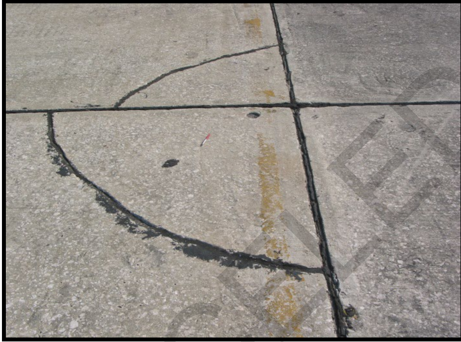
Figure B-6 Medium-Severity Corner Break
