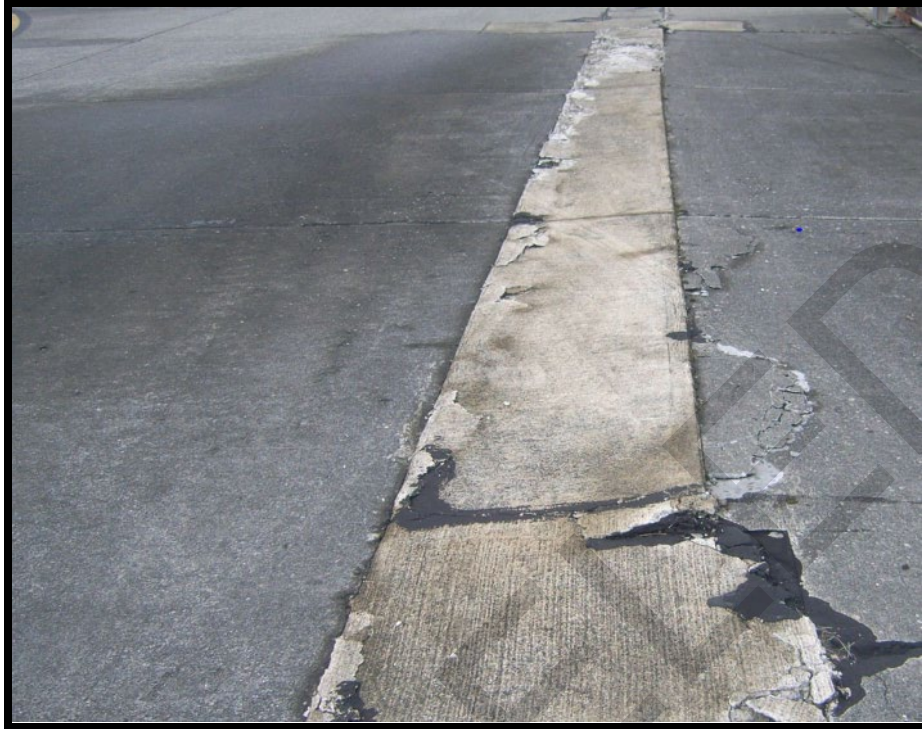
Figure B-2 Low-Severity Blowup
