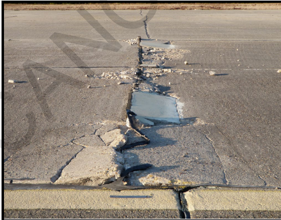
Figure B-4 High-Severity Blowup
