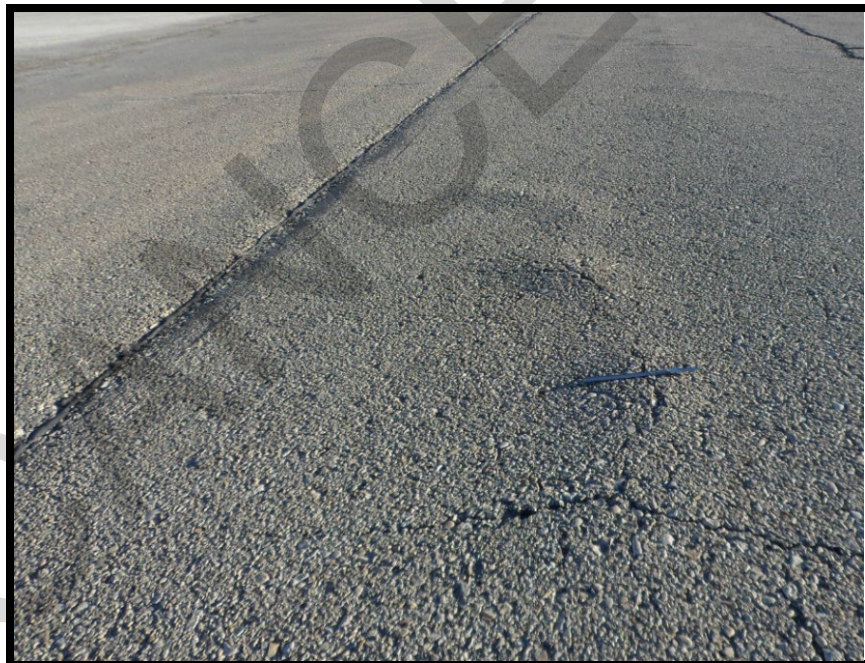
Figure A-51 Low-Severity Swell
