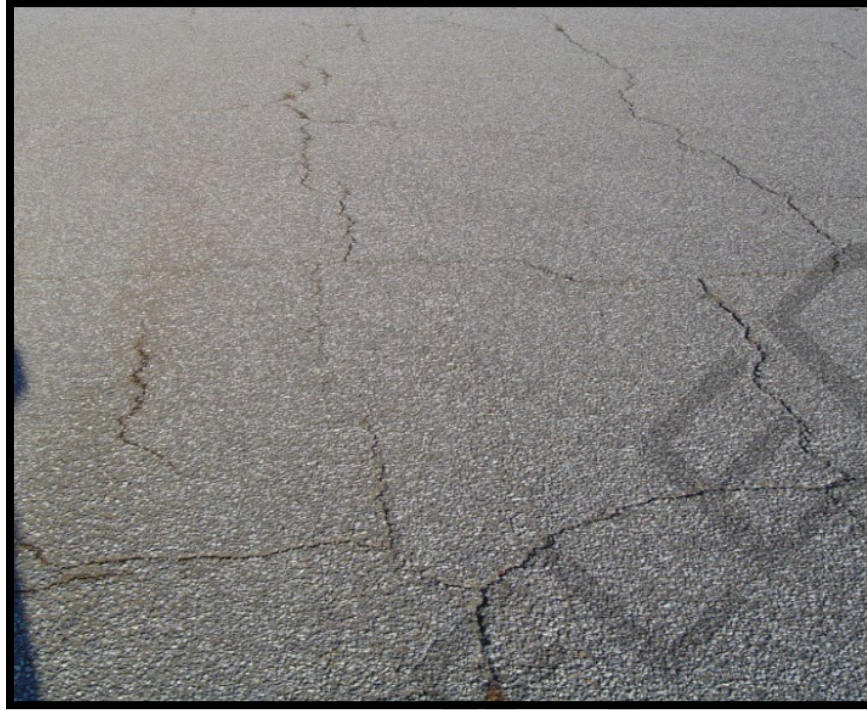
Figure A-10 High-Severity Block Cracking
