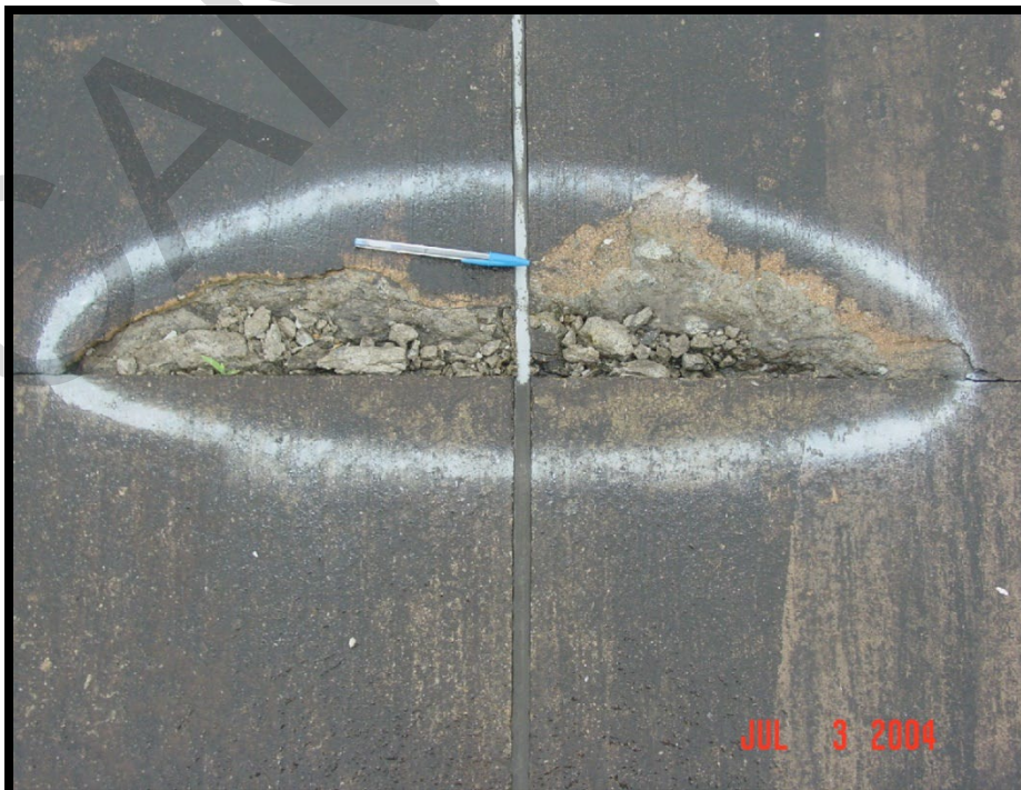
Figure B-40 High-Severity Joint Spall
