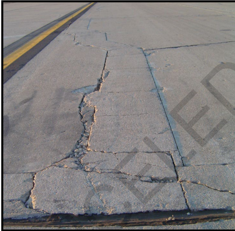
Figure B-23 High Severity Large Patch
