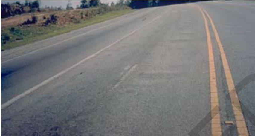
Figure A-14 Medium-Severity Corrugation
