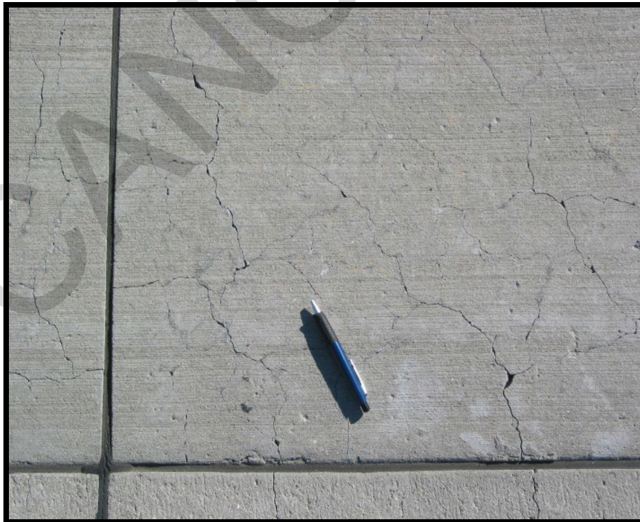
Figure B-45 Medium-Severity ASR
