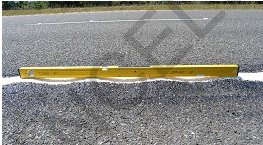
Figure A-14 Medium-Severity Corrugation
