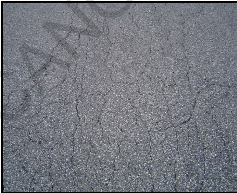
Figure A-2 Medium-Severity Alligator Cracking
