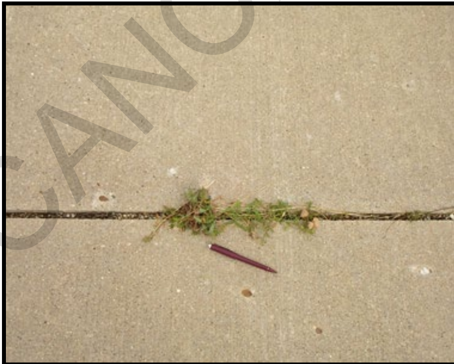
Figure B-17 High-Severity Joint Seal Damage
