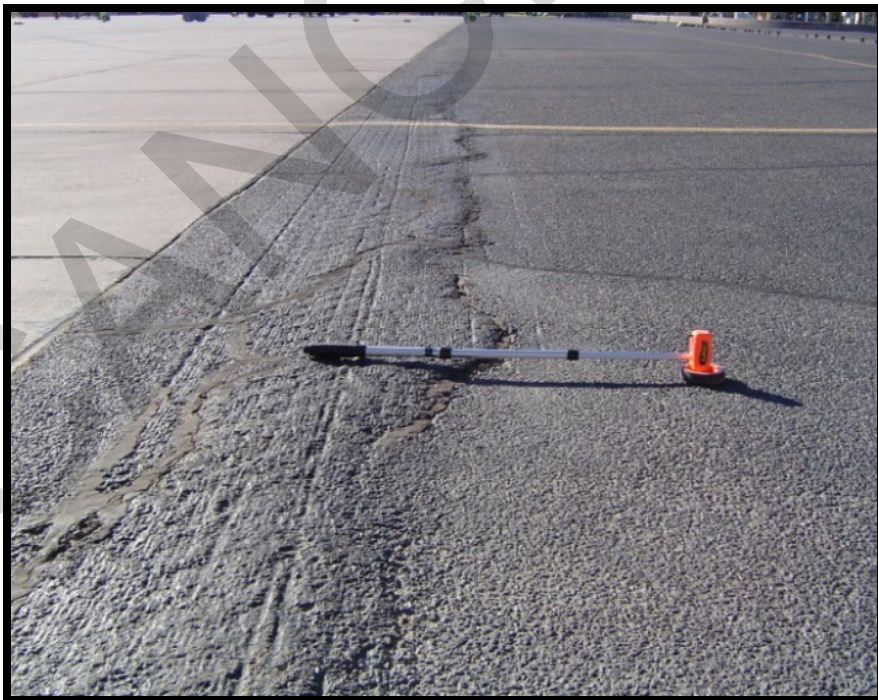
Figure A-48 Medium-Severity Shoving
