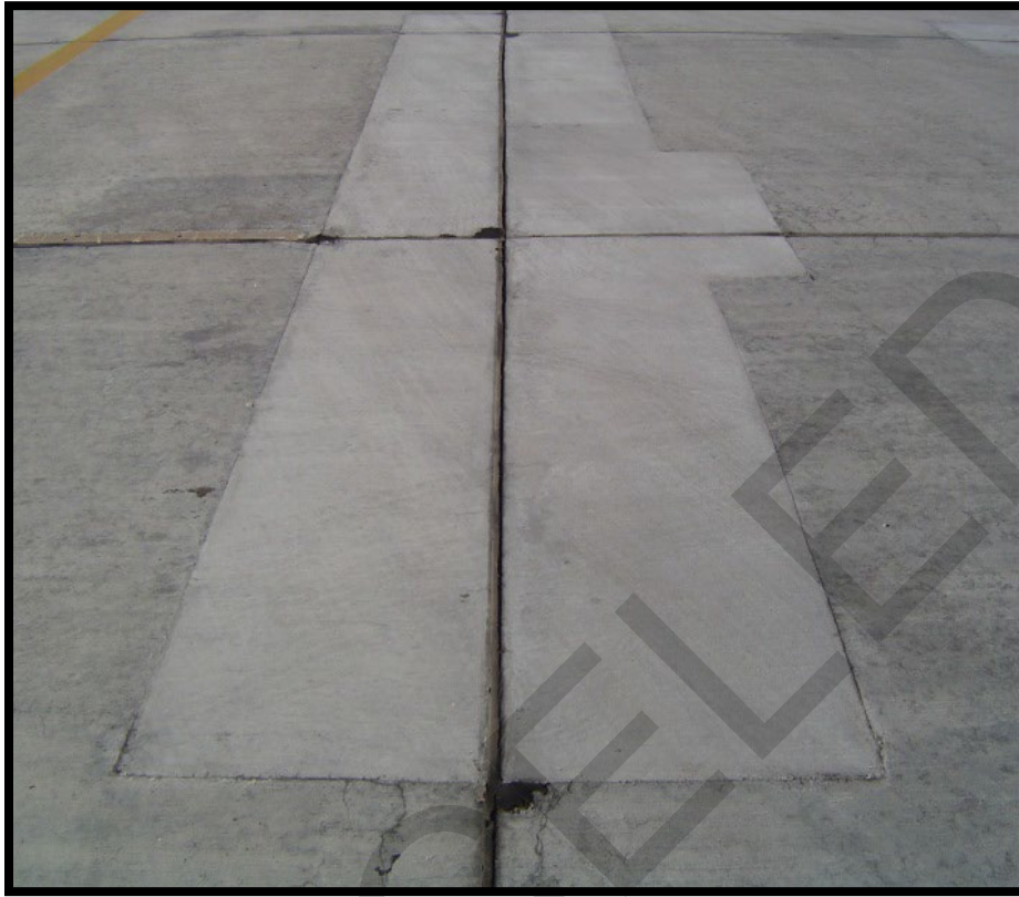
Figure B-22 Medium-Severity Large Patch
