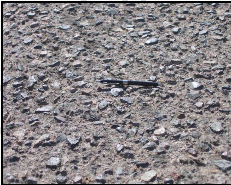
Figure A-56 High-Severity Weathering
