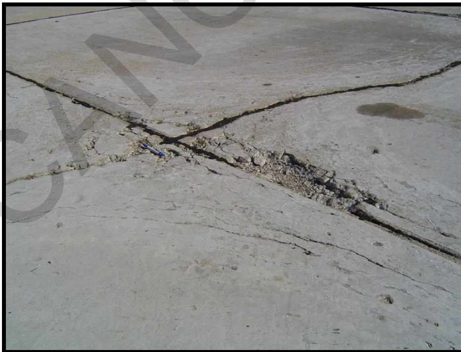
Figure B-14 High-Severity “D” Cracking
