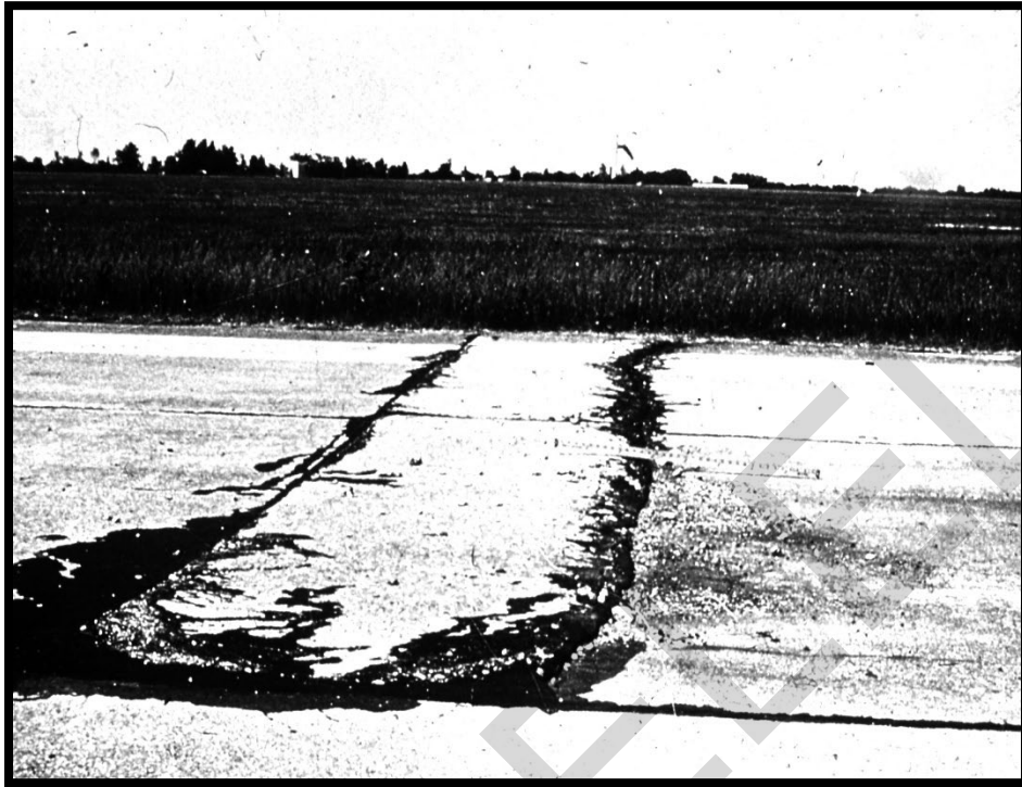
Figure B-4 High-Severity Blowup
