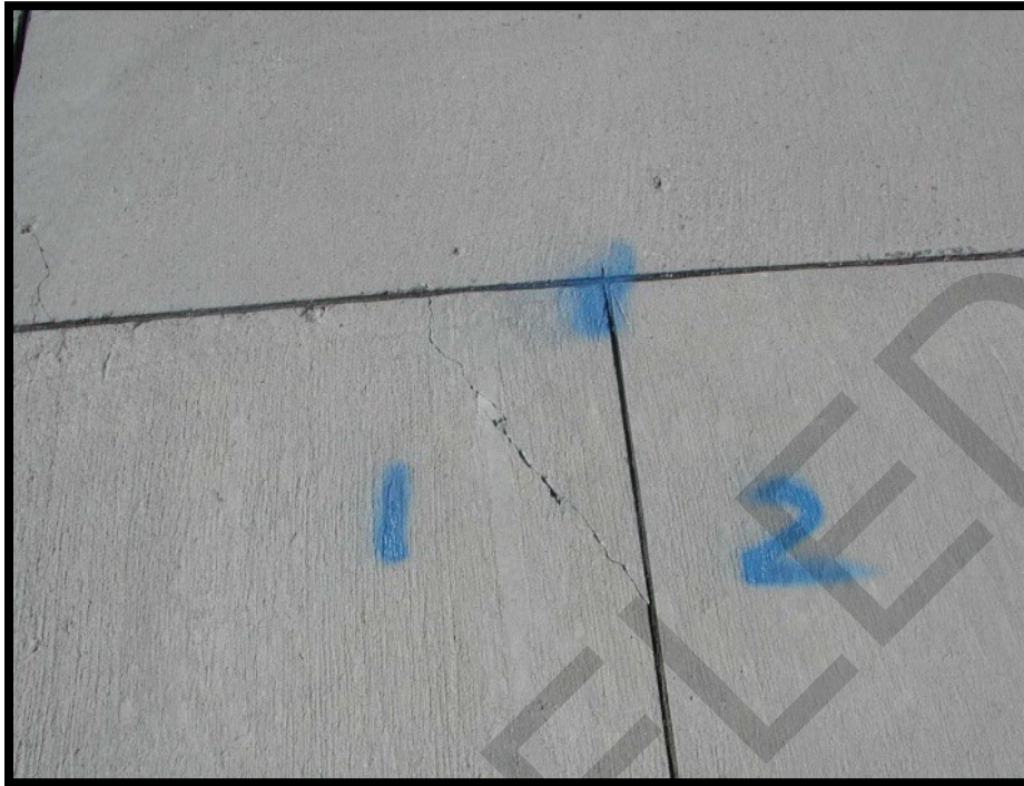
Figure B-42 Medium-Severity Corner Spall
