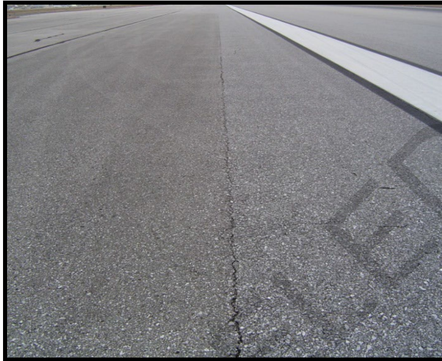
Figure A-25 Medium-Severity L&T Cracking
