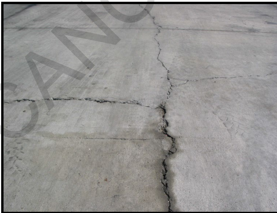
Figure B-35 High-Severity Shattered Slab/Intersecting Cracks
