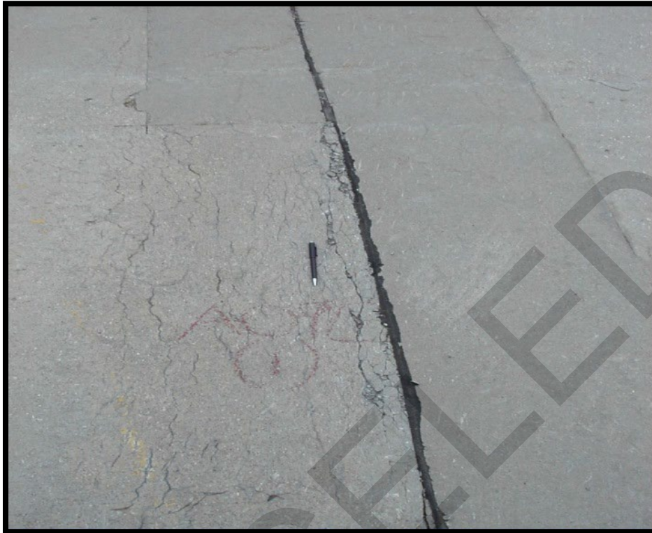
Figure B-14 High-Severity “D” Cracking
