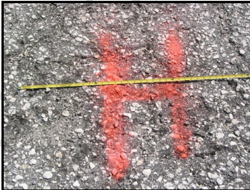
Figure A-38 High-Severity Raveling (Dense Mix)
