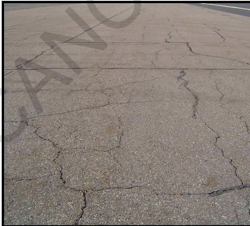
Figure A-8 Medium-Severity Block Cracking
