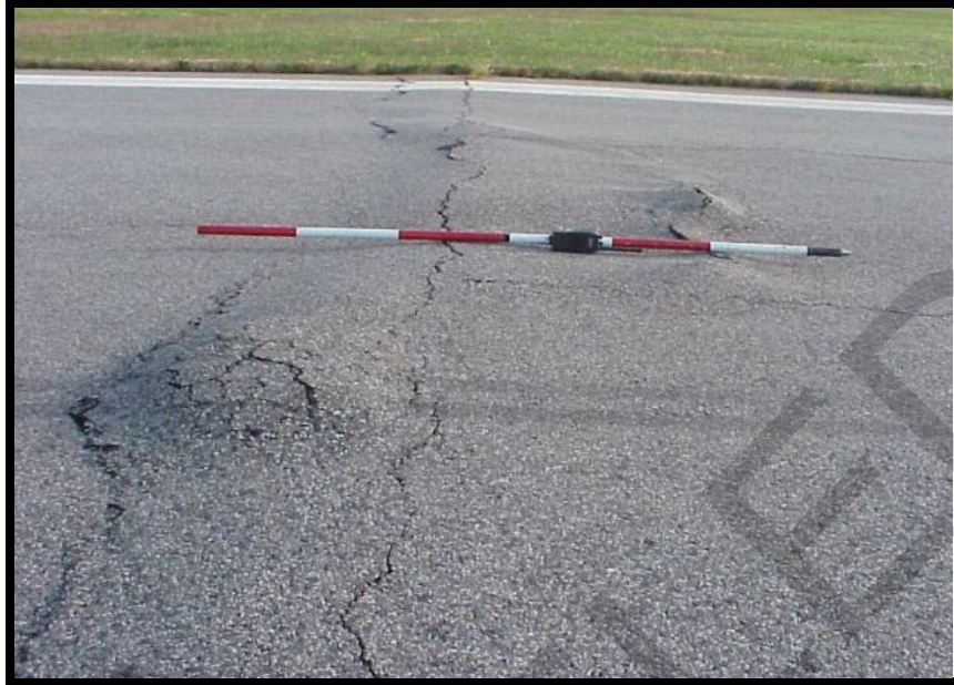
Figure A-53 High-Severity Swell
