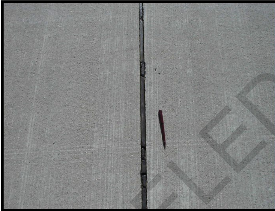
Figure B-17 High-Severity Joint Seal Damage
