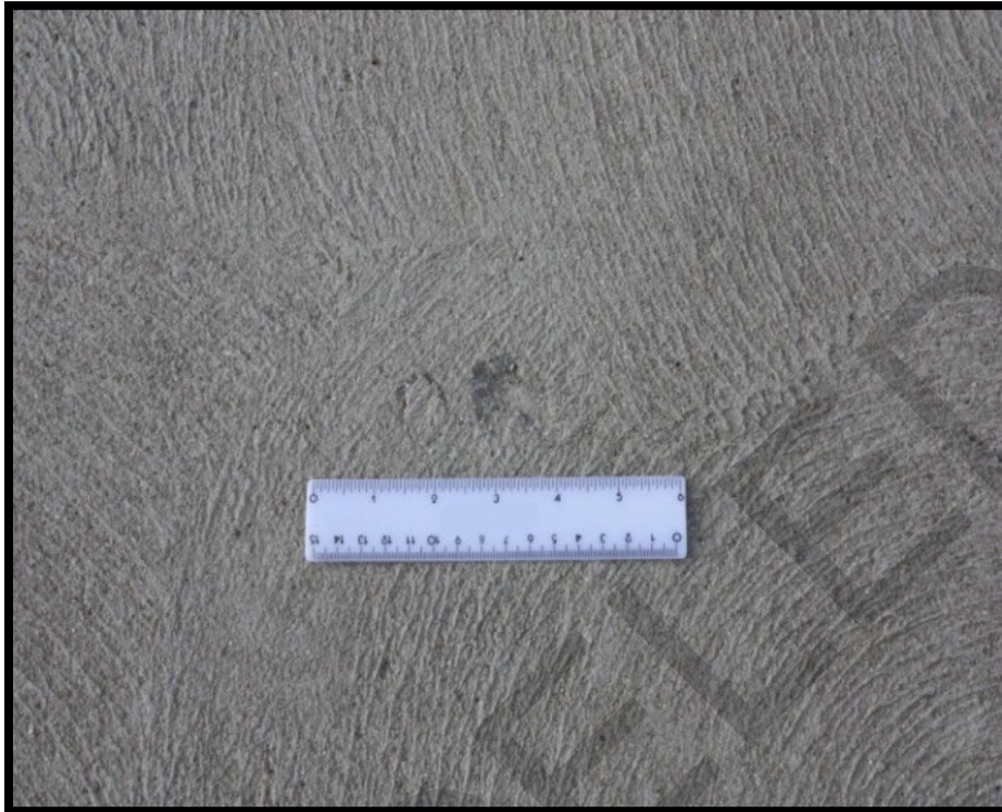
Figure B-28 Medium-Severity Scaling
