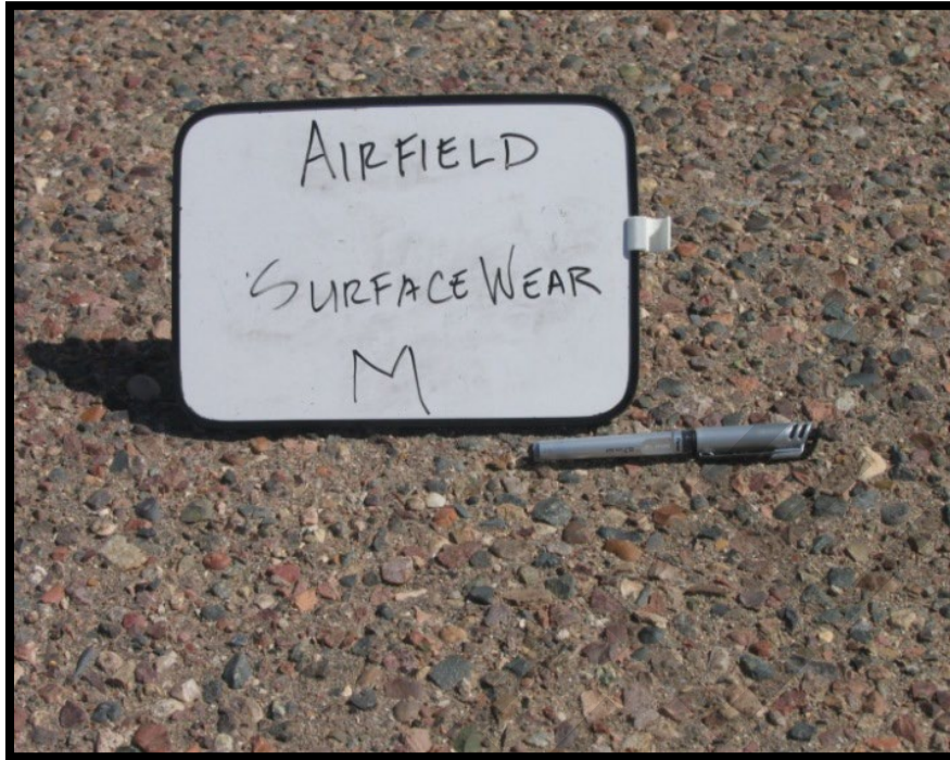
Figure A-56 High-Severity Weathering
