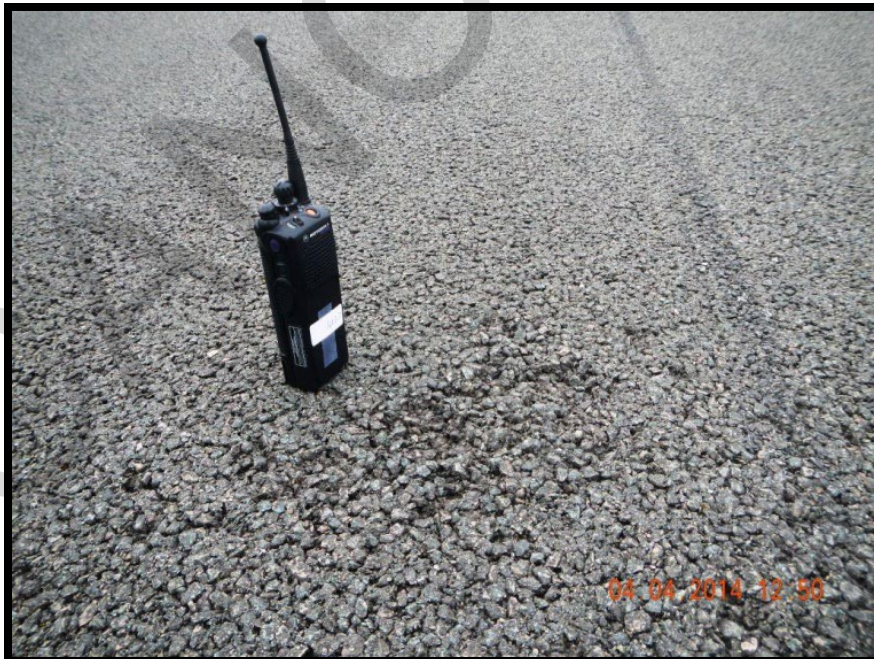
Figure A-44 Medium-Severity Raveling (PFC)
