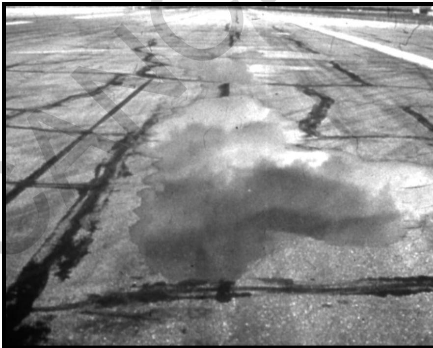
Figure A-18 High-Severity Depression
