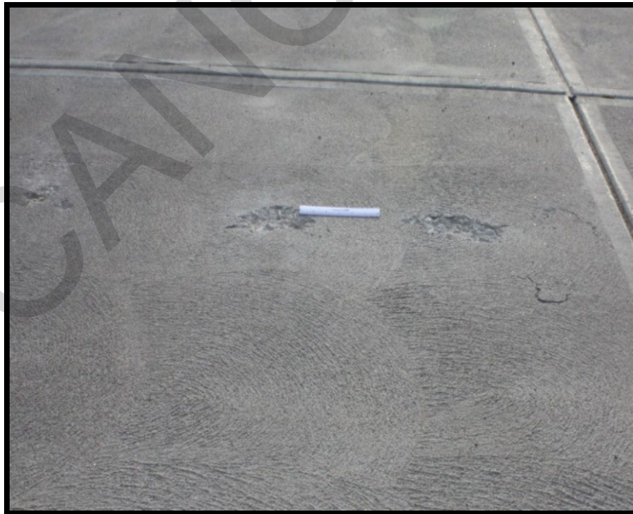
Figure B-28 Medium-Severity Scaling
