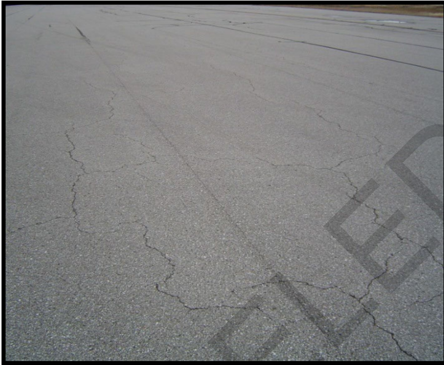
Figure A-8 Medium-Severity Block Cracking
