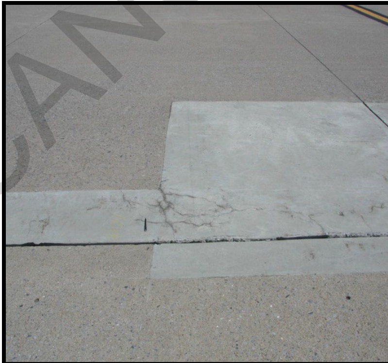
Figure B-22 Medium-Severity Large Patch
