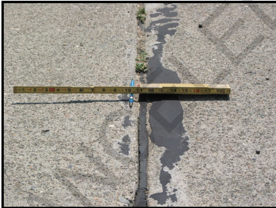
Figure B-30 Low-Severity Settlement or Faulting
