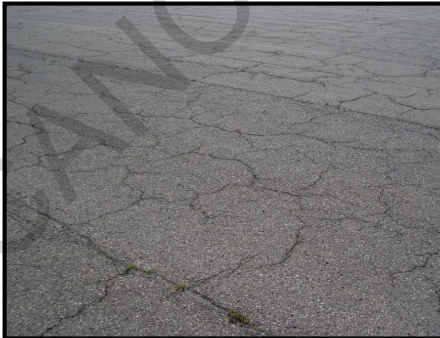
Figure A-10 High-Severity Block Cracking
