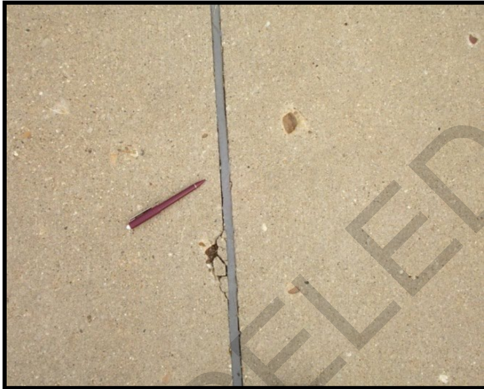
Figure B-38 Medium-Severity Joint Spall
