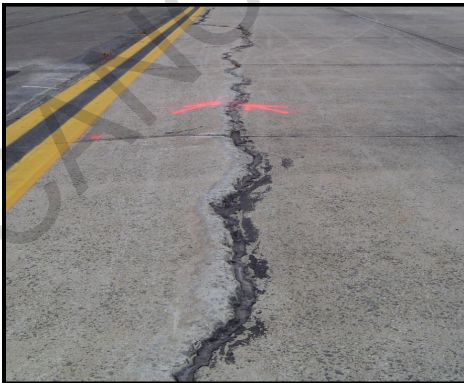
Figure B-2 Low-Severity Blowup
