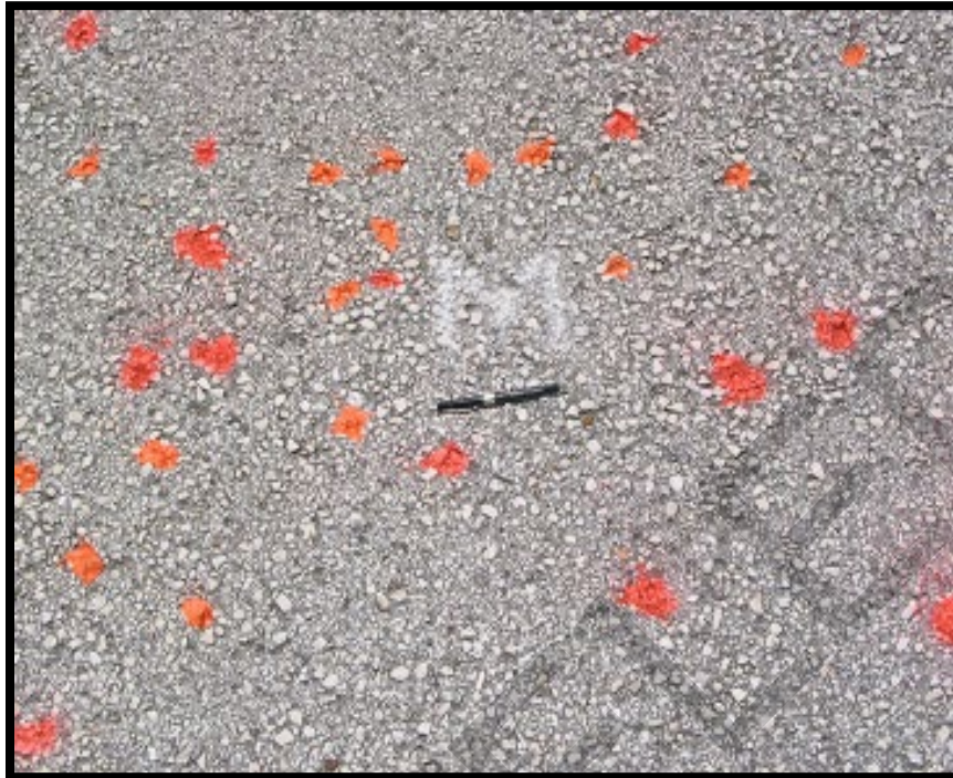
Figure A-38 High-Severity Raveling (Dense Mix)
