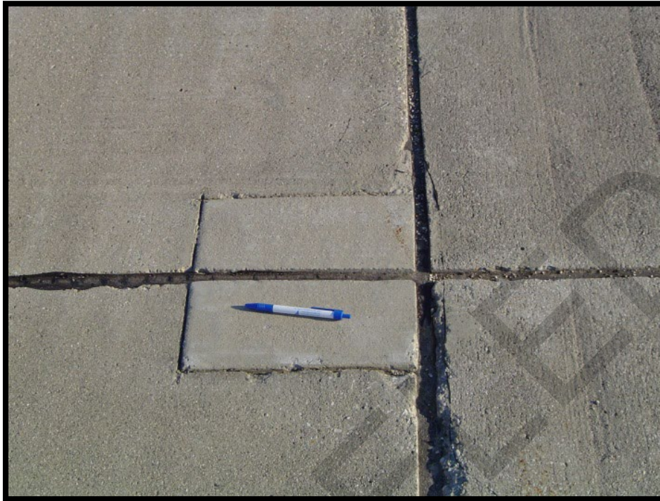
Figure B-19 Medium-Severity Small Patch
