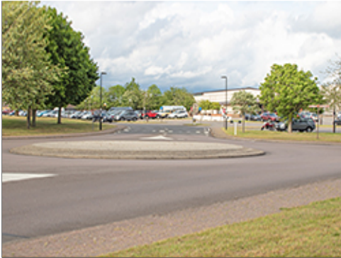
Central Paved Island
