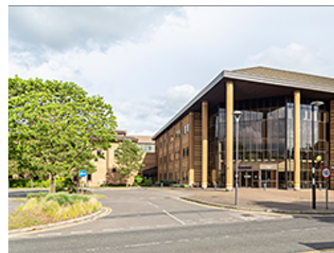
Intersection Adjacent to Group 1
