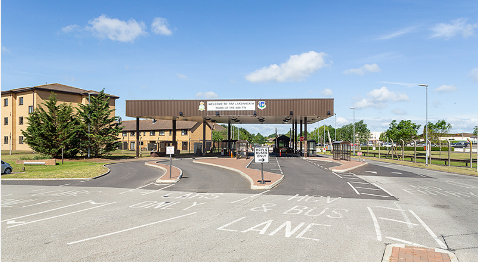
Main Gate at Brandon Road
