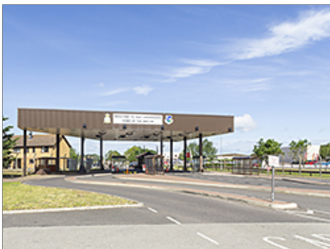
Arterial at Main Gate
