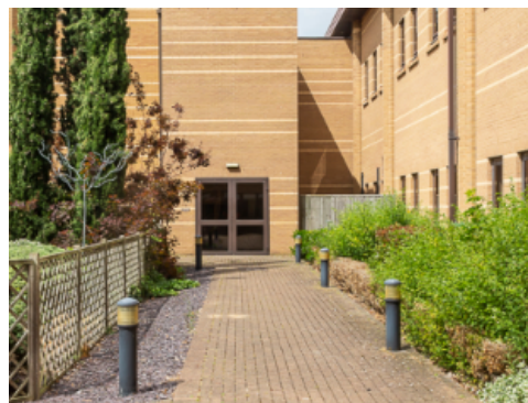
Bollard Lights at Hospital
