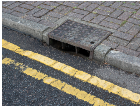
Storm Drain at Street
