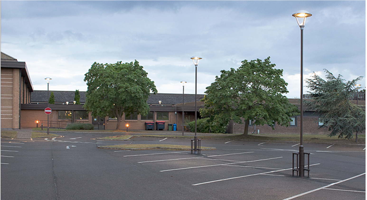
Standard Lighting at Parking Lot
