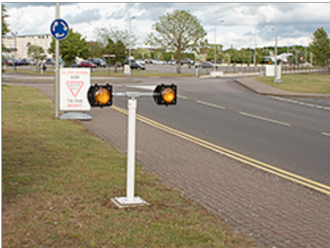
Signal at Special Intersection
