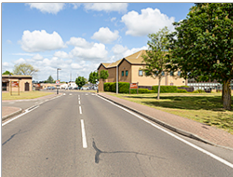
Collector with Attached Sidewalk
