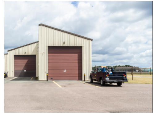
Parking Adjacent to Workspace
