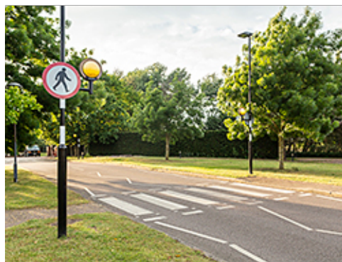
Painted Crosswalk and Markings
