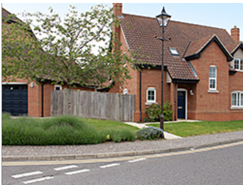
Street Elements in Group 4
