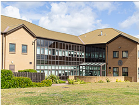
Curtain Wall Glazing Used as a Feature
