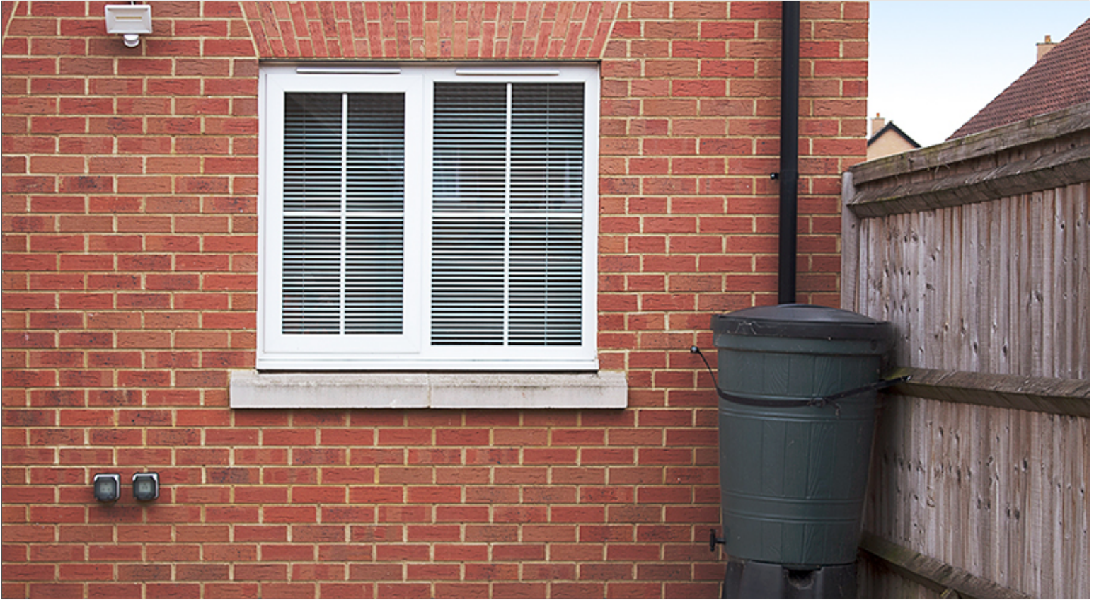
Rainbarrel Delays Release of Water
