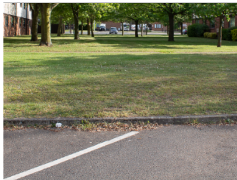
Concrete Curb at Grass
