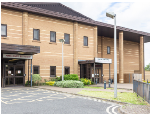
Lighting at Entry
