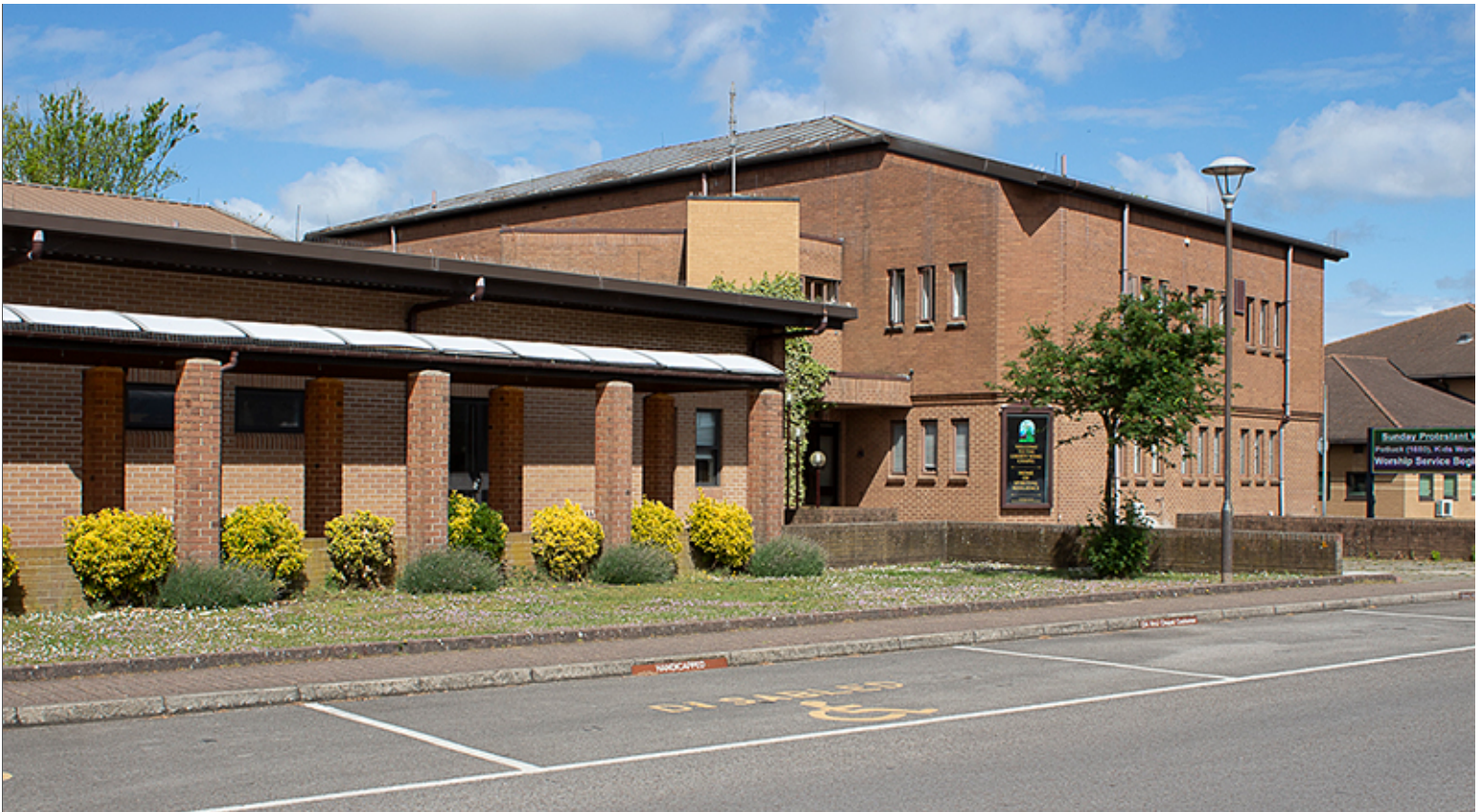
Parallel Parking at Building
