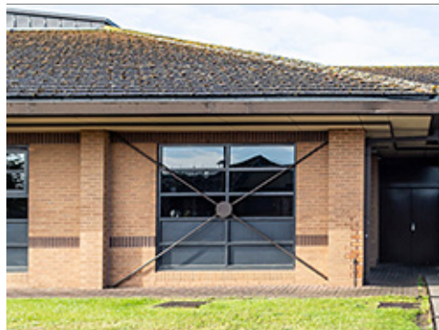
Exposed Structural Element
