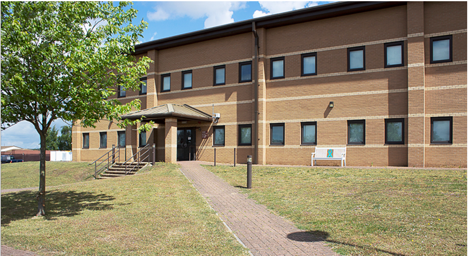
Ramp and Stair to Building
