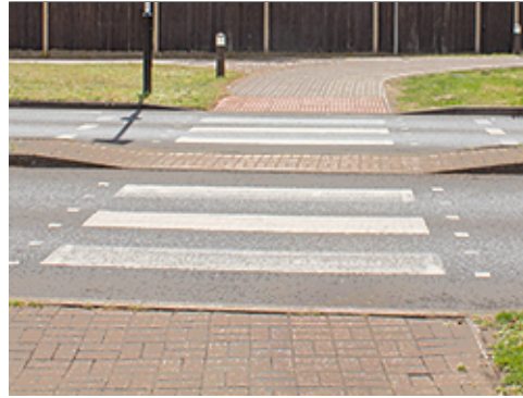
Curb Ramp at Crosswalk
